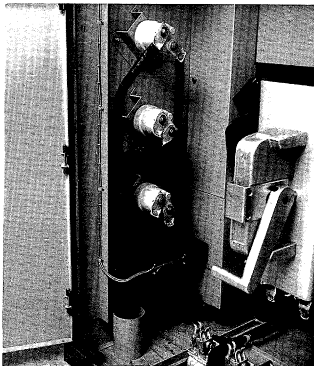
Fig. 78. Motor terminal and channel for control wiring in bottom compartment of one-high 34-inch enclosure.
