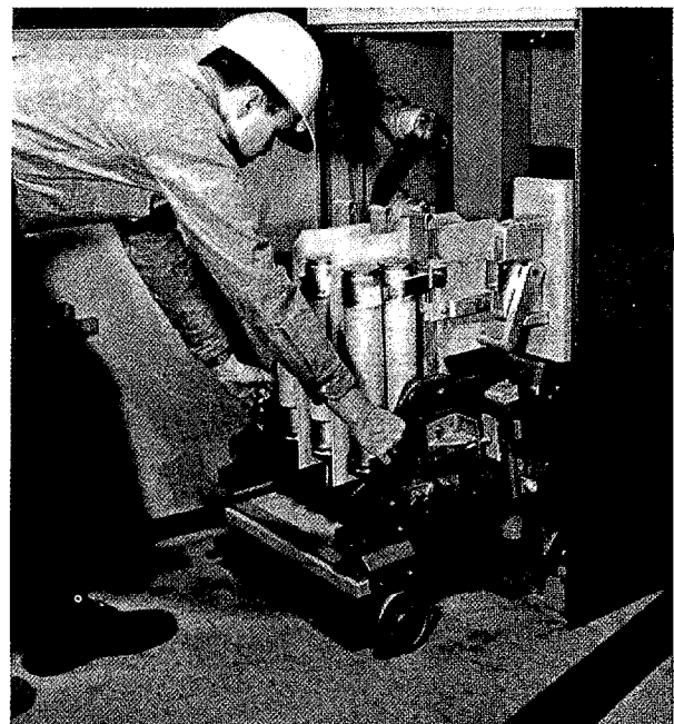
Fig. 26. Roll contactor out of enclosure.
