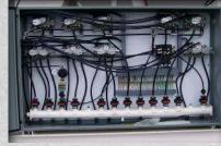
Enclosure for air valves with safety valves which isolate each solenoid for quick repair if needed. Solenoids are wired to central terminal to ease of service.
