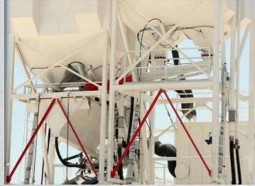
The cement batcher is equipped with an air slide discharge system which allows for a quick and even discharge. Both the cement batcher and auxiliary silo air slide are supplied air from a 5HP aeration blower.
