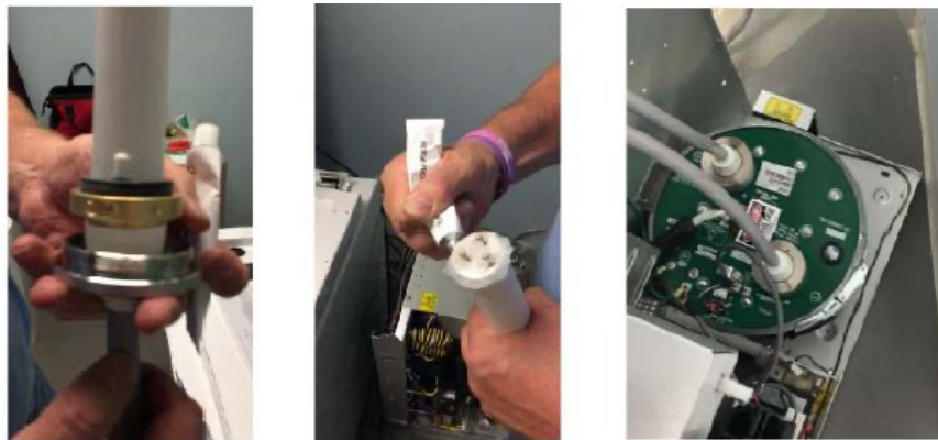
Figure 5: Connecting the high tension cables to the generator
