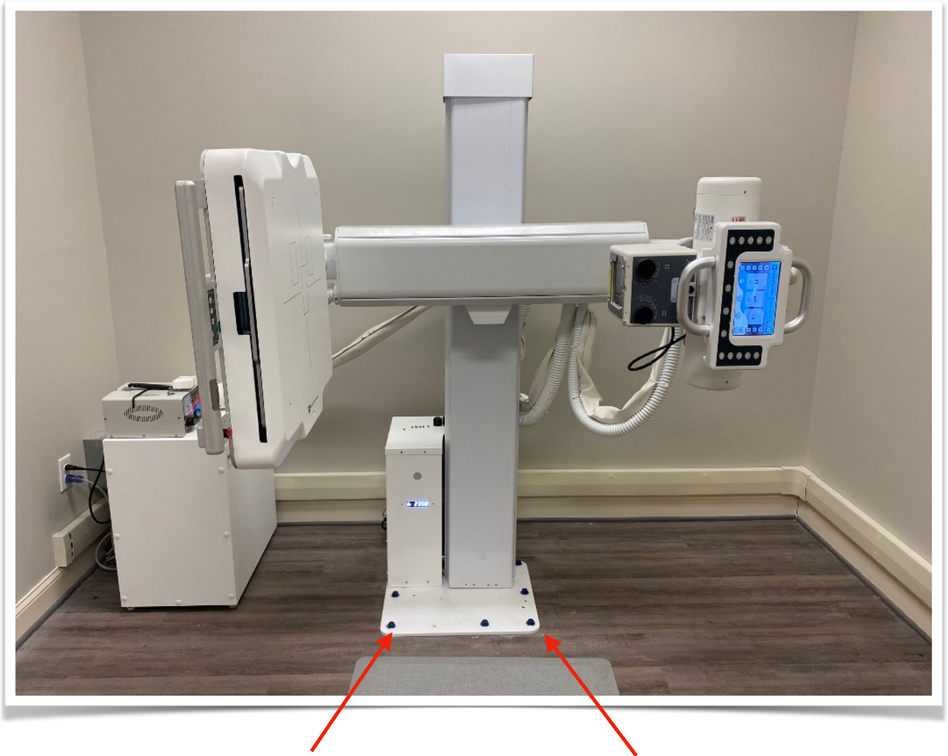
Figure 2: anchoring the MX40 to the floor
