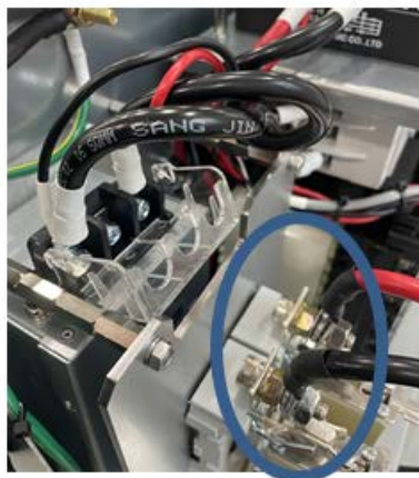
Connect the power cable of Generator
