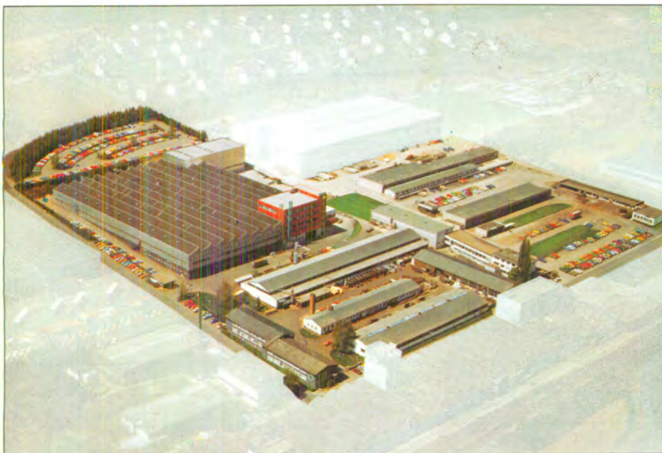
Aerial photograph of our factory in Tauberbischofsheim (publication approved by Reg. Präs., No. 9/54 571)
