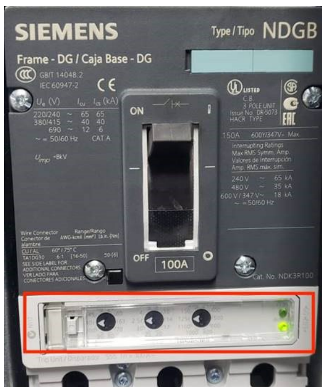
Figure 1-4: Printer Main AC Breaker
