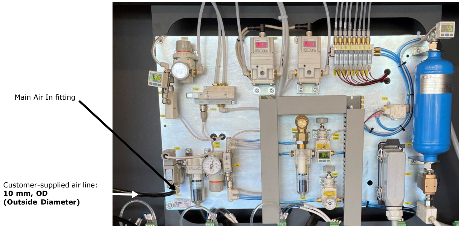
Figure 1-16: Main Air Panel - Air input location
