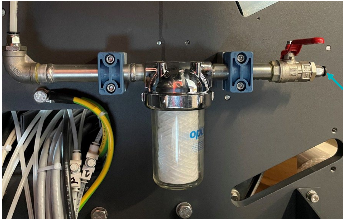
Figure 1-17: Main Water Supply Connection
