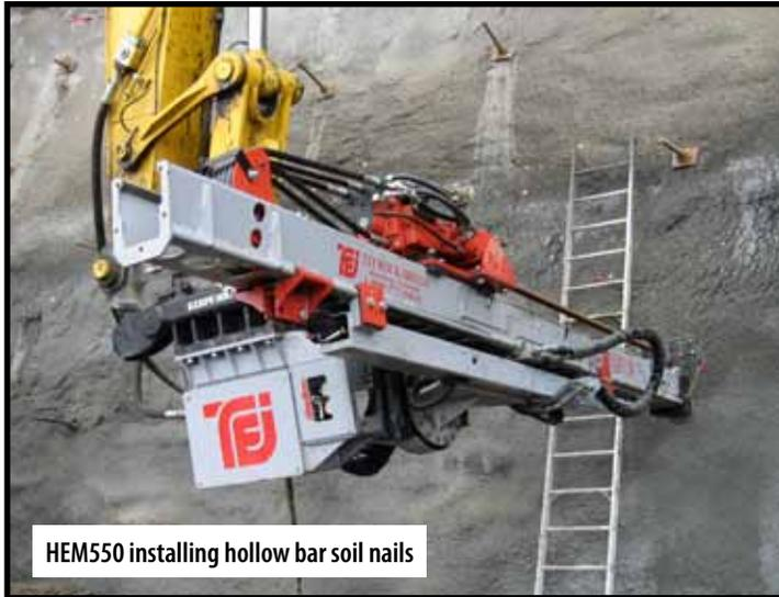
HEM550 installing hollow bar soil nails
