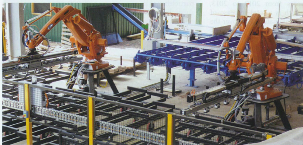
■ An aerial shot of the system during installation.
