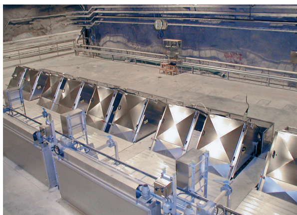
Meva Rotoscreen in a WWTP
