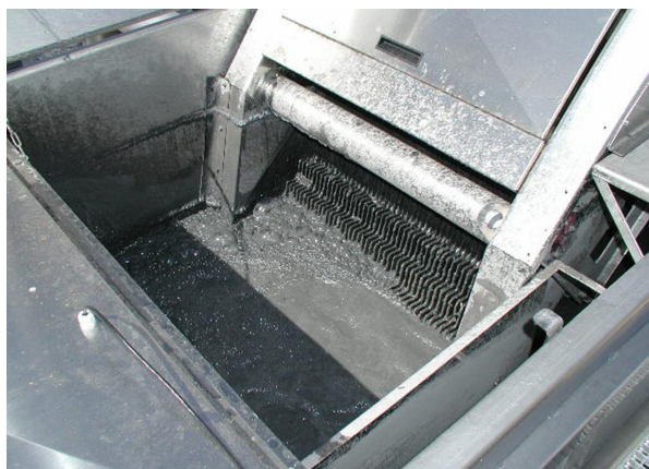
Meva Rotoscreen in a tank
