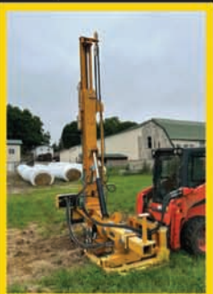
2022 Rhino Solar Pro Pile Driver - Hillpoint, WI
