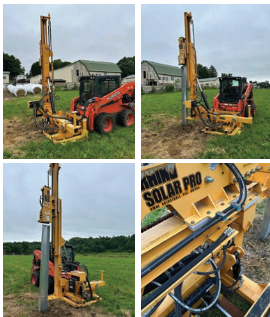
2022 Rhino Solar Pro Pile Driver
