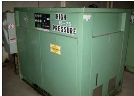
SULLAIR ROTARY SCREW AIR COMPRESSOR #16-75
