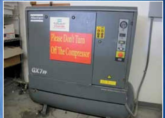
Atlas Copco Rotary Screw Air Compressor Model GX7-FF
