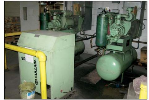
VIEW OF SULLAIR ROTARY SCREW AIR
