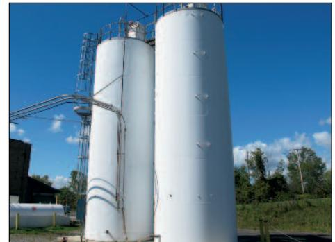
(2) 16' DIA. X 32'T STORAGE SILOS, WITH 1,000-LB. VOLUMETRIC WEIGH SCALE
