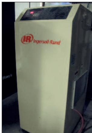
Ingersoll Rand Compressed Air Dryer Model NVC200A200,
