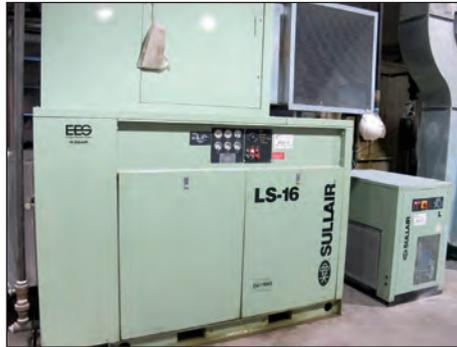
SULLAIR ROTARY SCREW AIR COMPRESSOR MODEL LS-16
