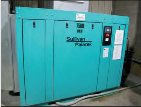
SULLIVAN PALATEK 75 HP ROTARY SCREW AIR COMPRESSOR MODEL 75UD-VFD
