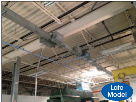
View of ELECTRICAL BUSS BAR
