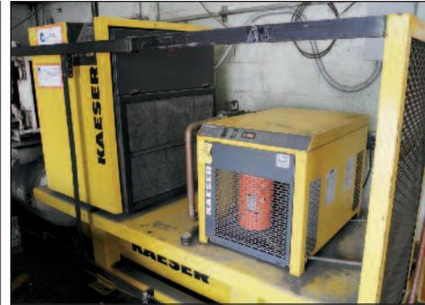
Kaiser 20 HP Rotary Screw Air Compressor Model SK25
