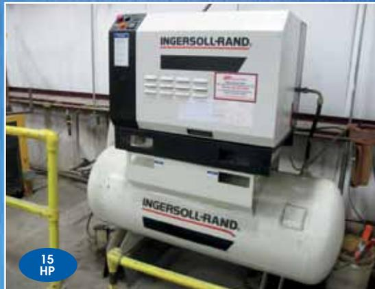
INGERSOLL RAND ROTARY SCREW AIR COMPRESSOR
