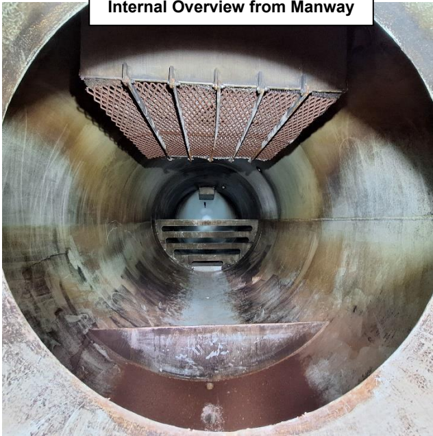
Internal Overview from Manway
