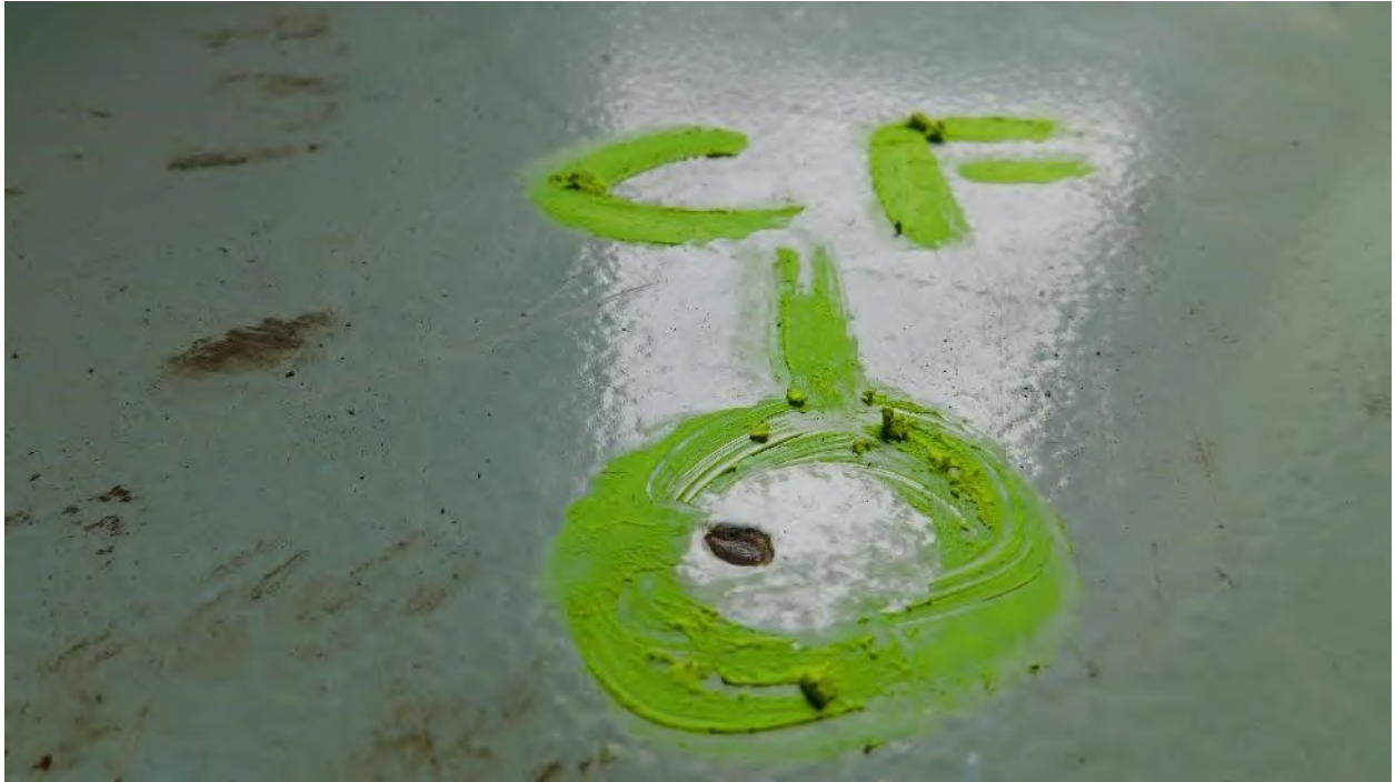
Photograph 23: Bottom Plate Coating Failure Detail
