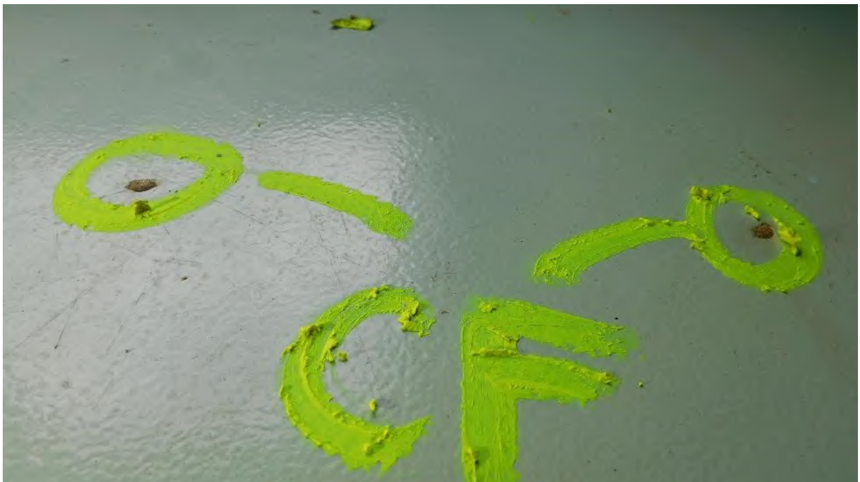
Photograph 24: Bottom Plate Coating Failure Detail
