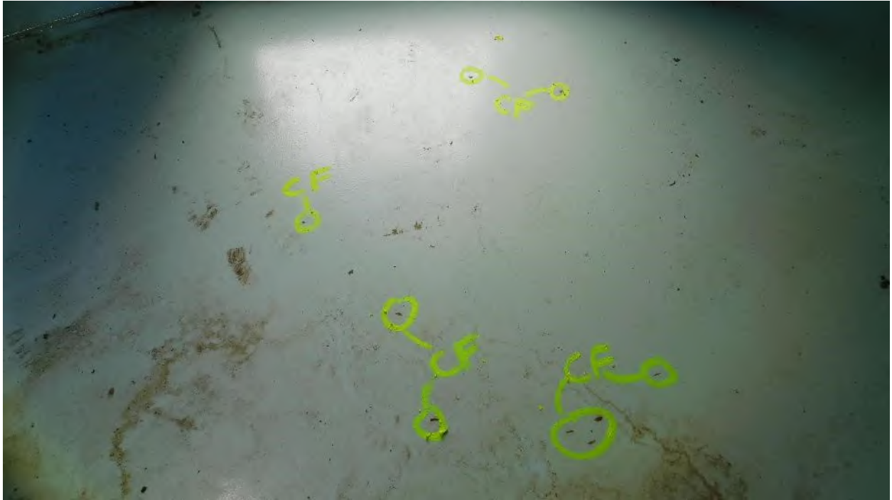
Photograph 21: Bottom Plate Coating Failure Overview
