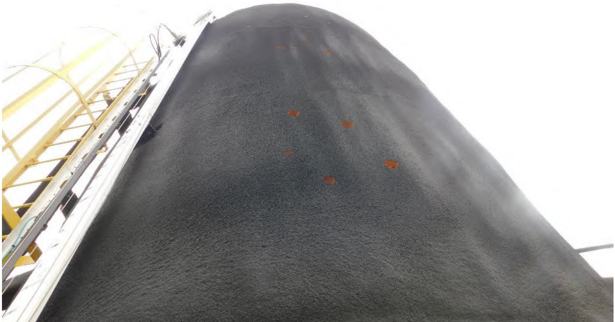
Photograph 38: External Shell Overview – General Minor Insulation Damage
