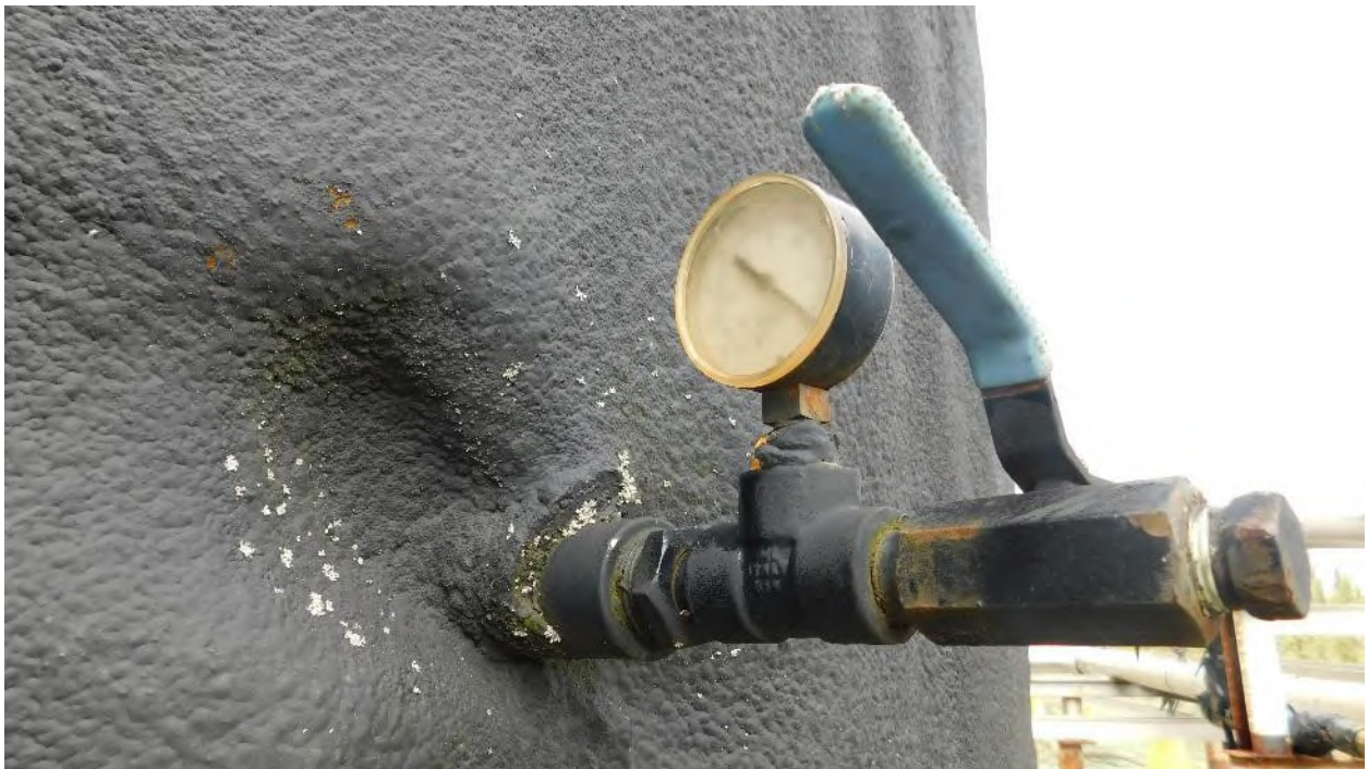
Photograph 48: 1" Threaded Pressure Gauge Nozzle
