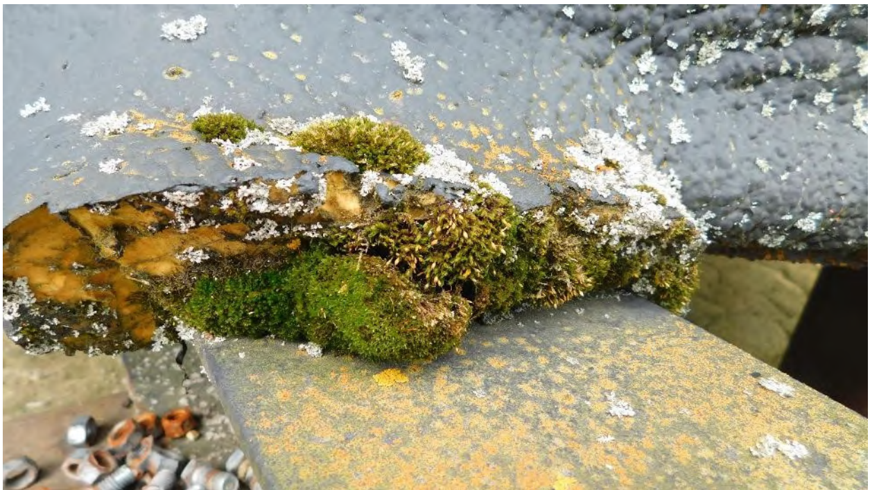
Photograph 18: Bottom Plate Projection – Moss Growth
