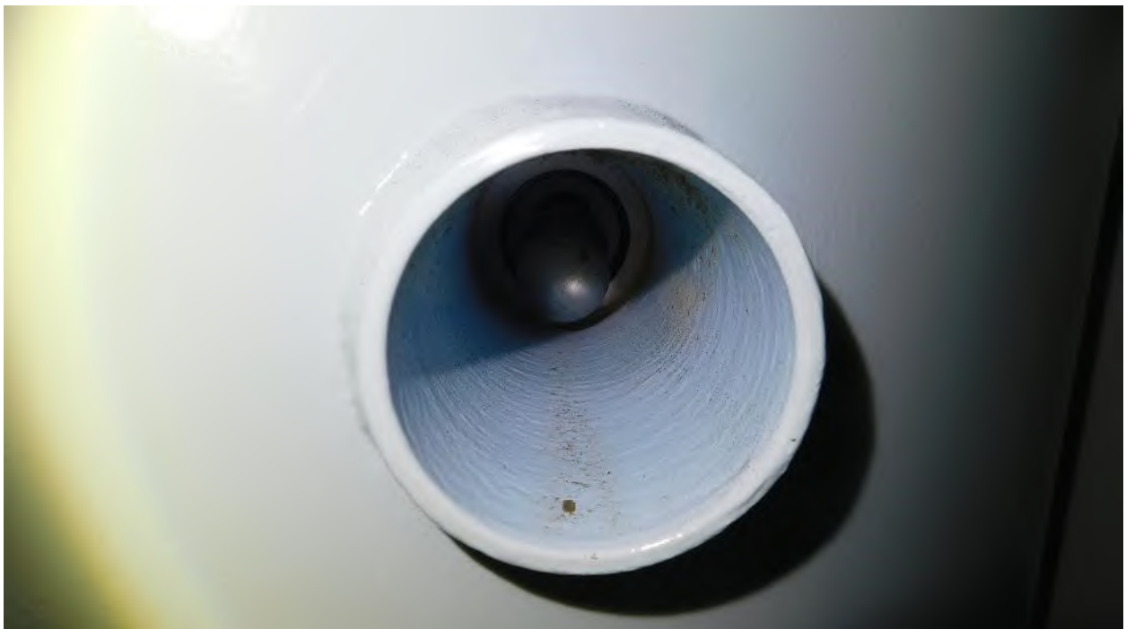
Photograph 60: 4" Internal Nozzle - EnviroVault
