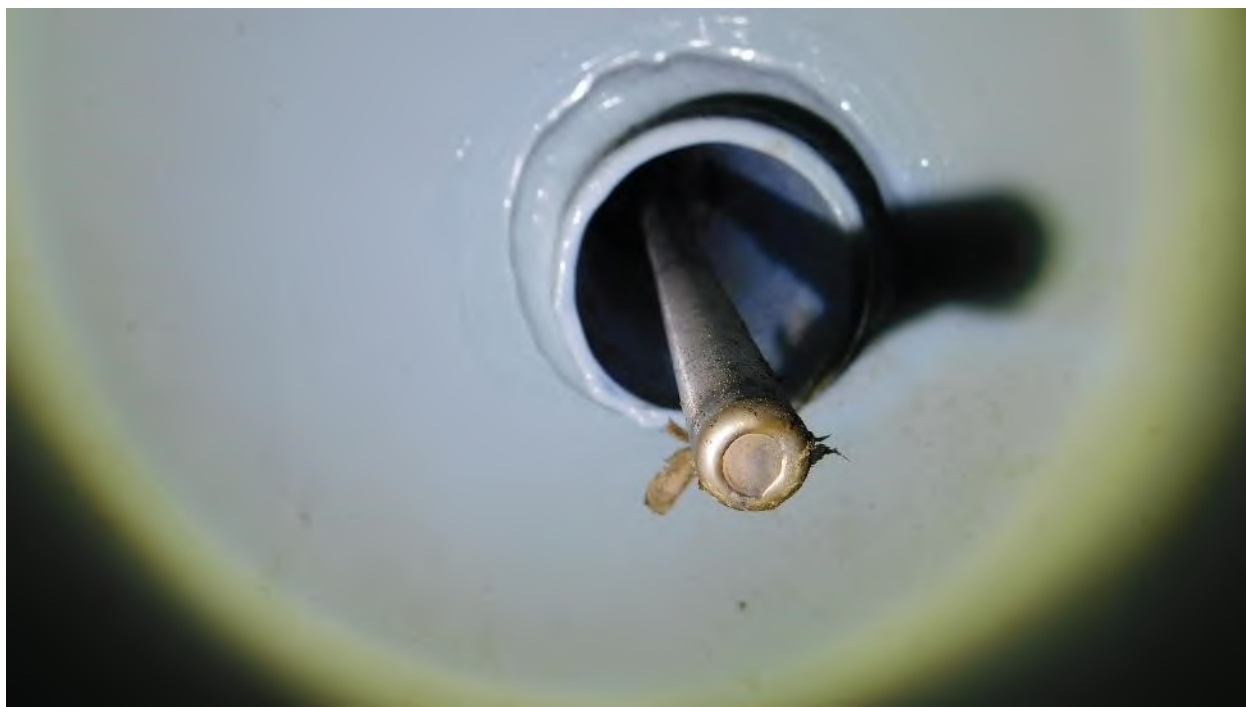
Photograph 61: 3" Internal Instrumentation Nozzle - EnviroVault
