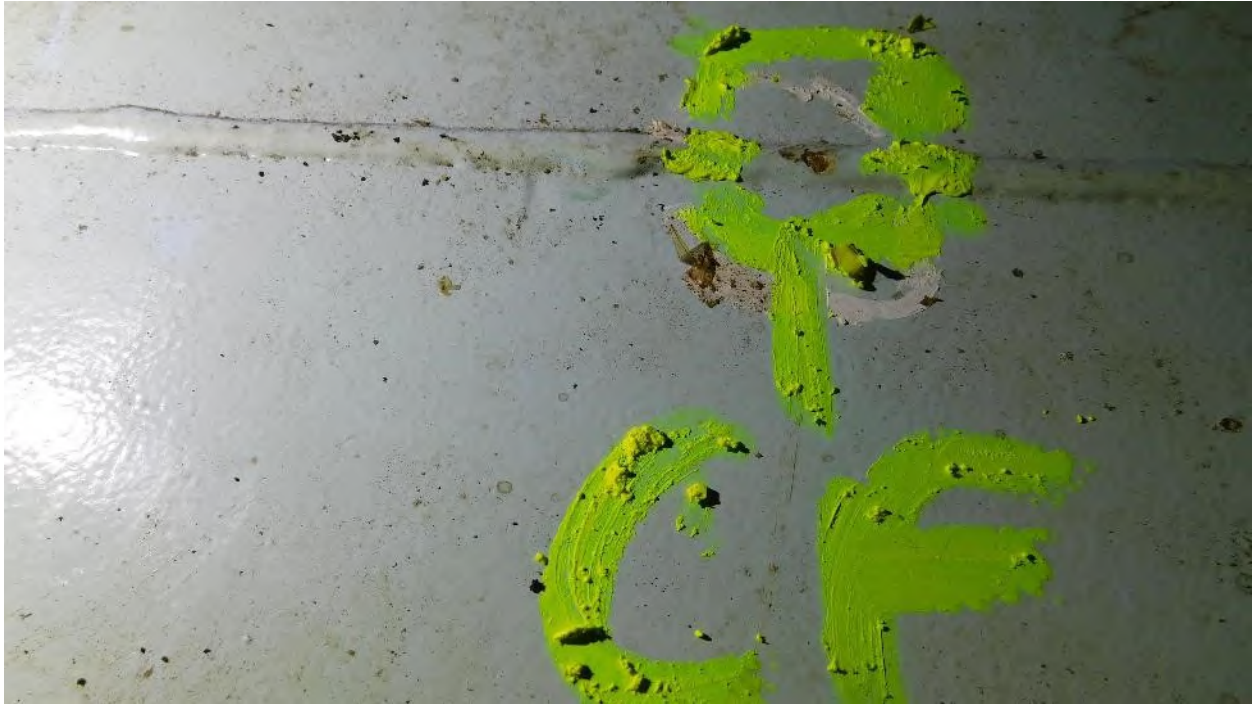
Photograph 29: Bottom Plate Weld Coating Failure Detail
