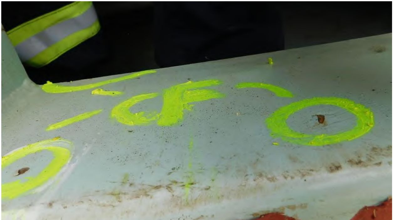
Photograph 56: Manway Coating Failure Detail
