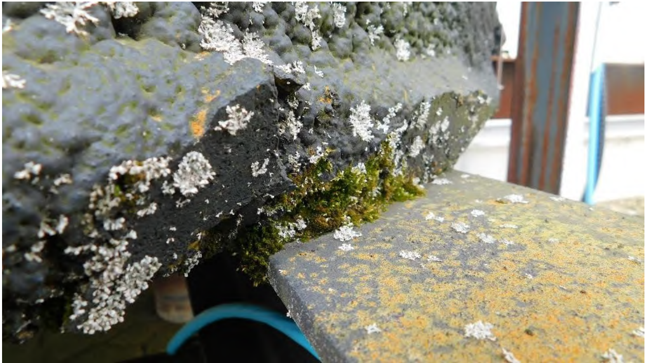
Photograph 17: Bottom Plate Projection – Moss Growth
