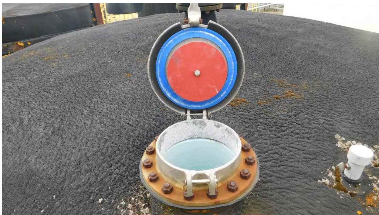
Photograph 67: Gauge Hatch Detail
