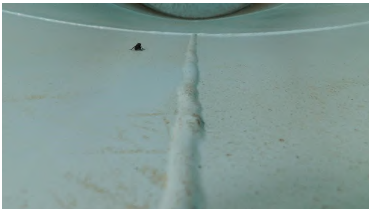
Photograph 43: Shell Butt Vertical Weld Profile
