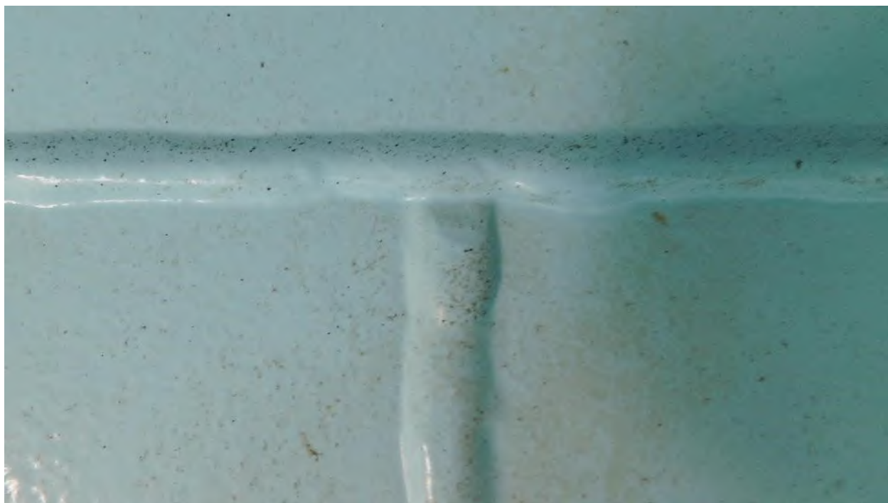
Photograph 44: Shell Butt Weld Detail
