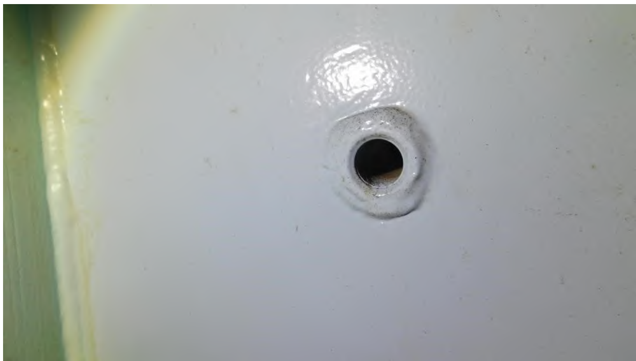
Photograph 57: 1" Threaded Nozzle
