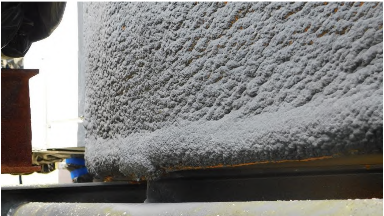
Photograph 16: Bottom Plate Projection Overview (Insulated)
