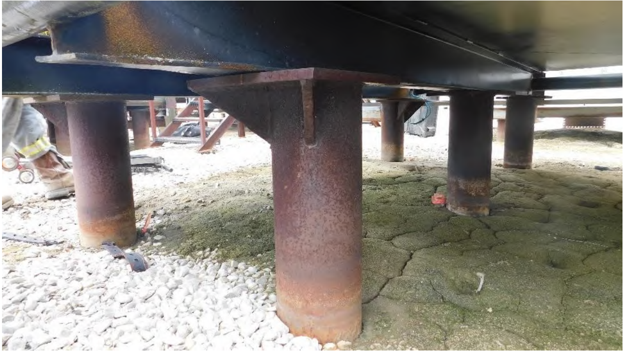
Photograph 15: Tank Resting on Piles and I Beam Structural Steel
