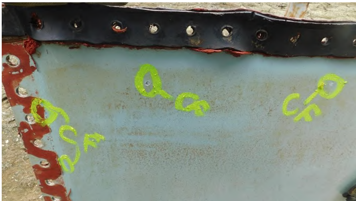
Photograph 63: Manway Cover – Coating Failure
