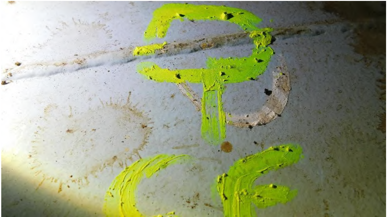
Photograph 27: Bottom Plate Weld Coating Failure Detail
