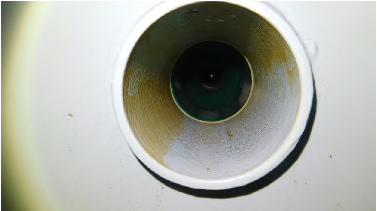
Photograph 59: 4" Internal Nozzle - EnviroVault
