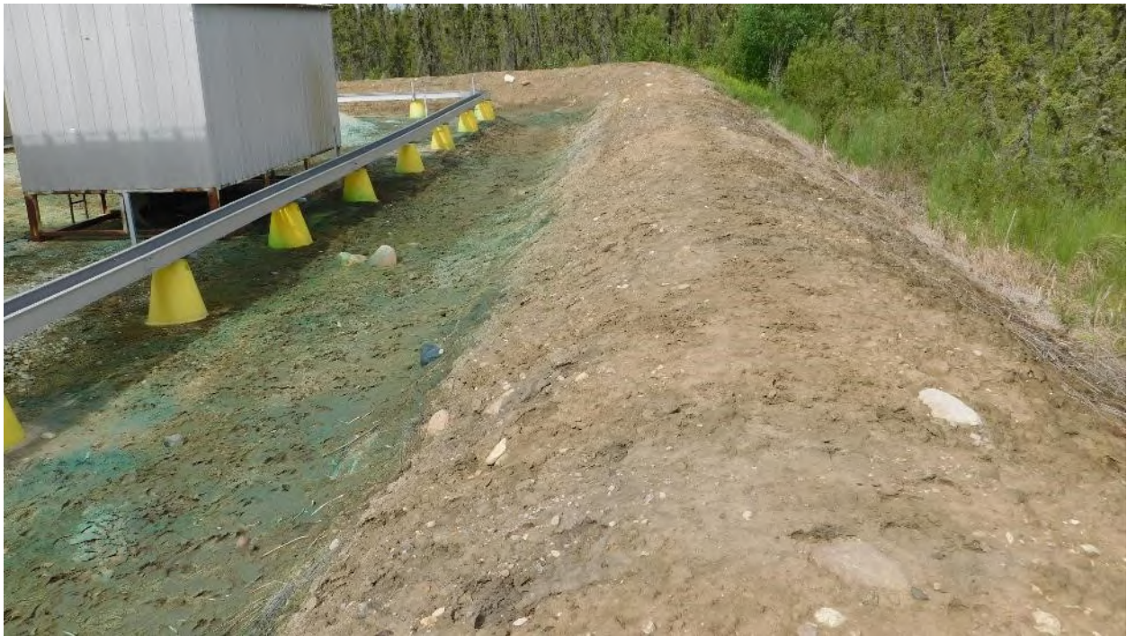
Photograph 6: Secondary Containment Sloped Wall Overview
