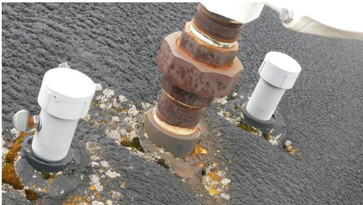
Photograph 70: Fixed Roof Gauge Board Threaded Nozzles – Moss Growth
