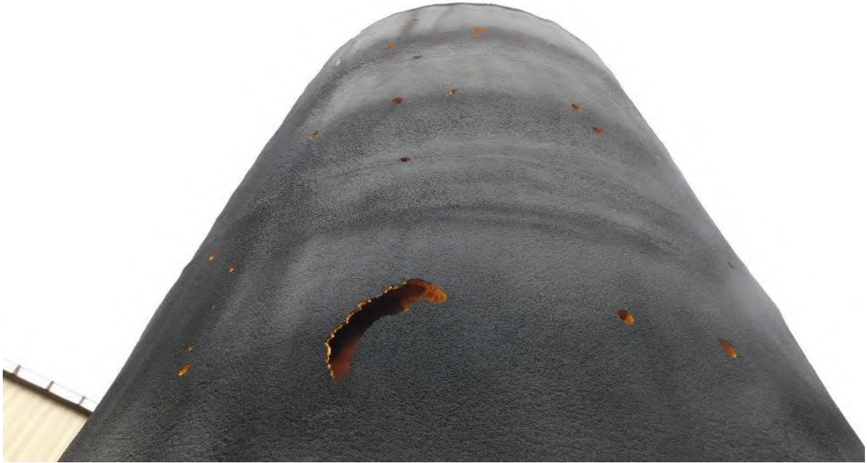
Photograph 34: External Shell Overview – General Minor Insulation Damage
