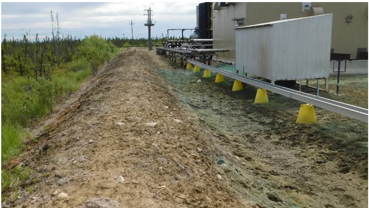
Photograph 9: Secondary Containment Sloped Wall Overview
