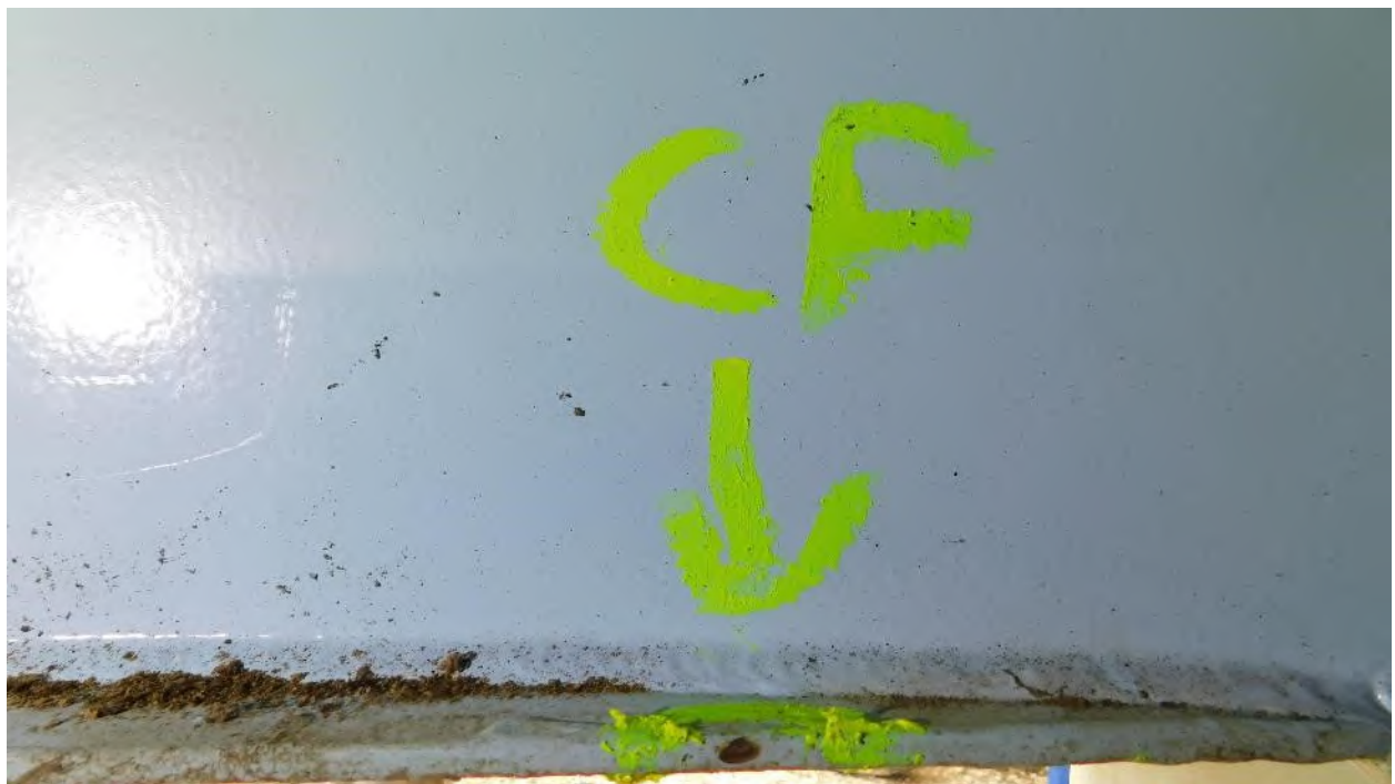
Photograph 54: Manway Coating Failure Detail
