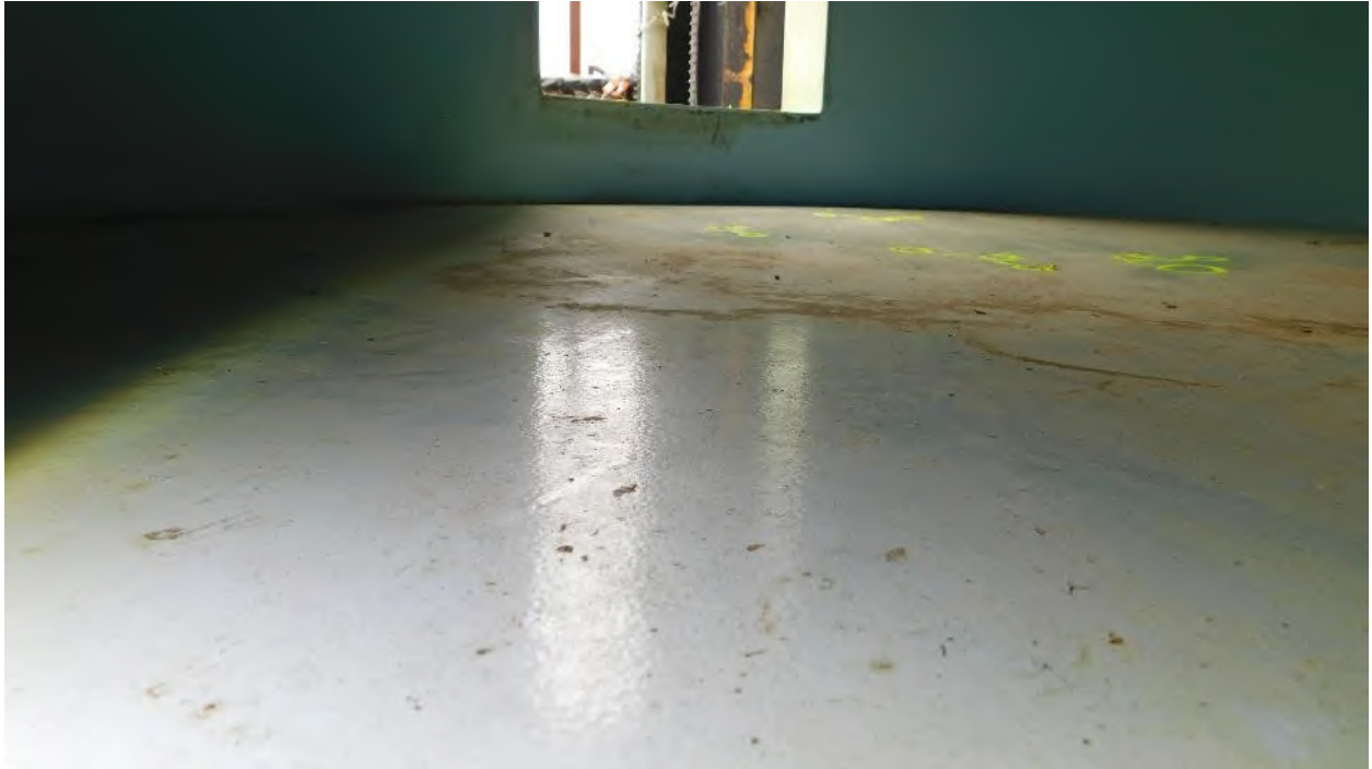
Photograph 31: Bottom Plate Profile
