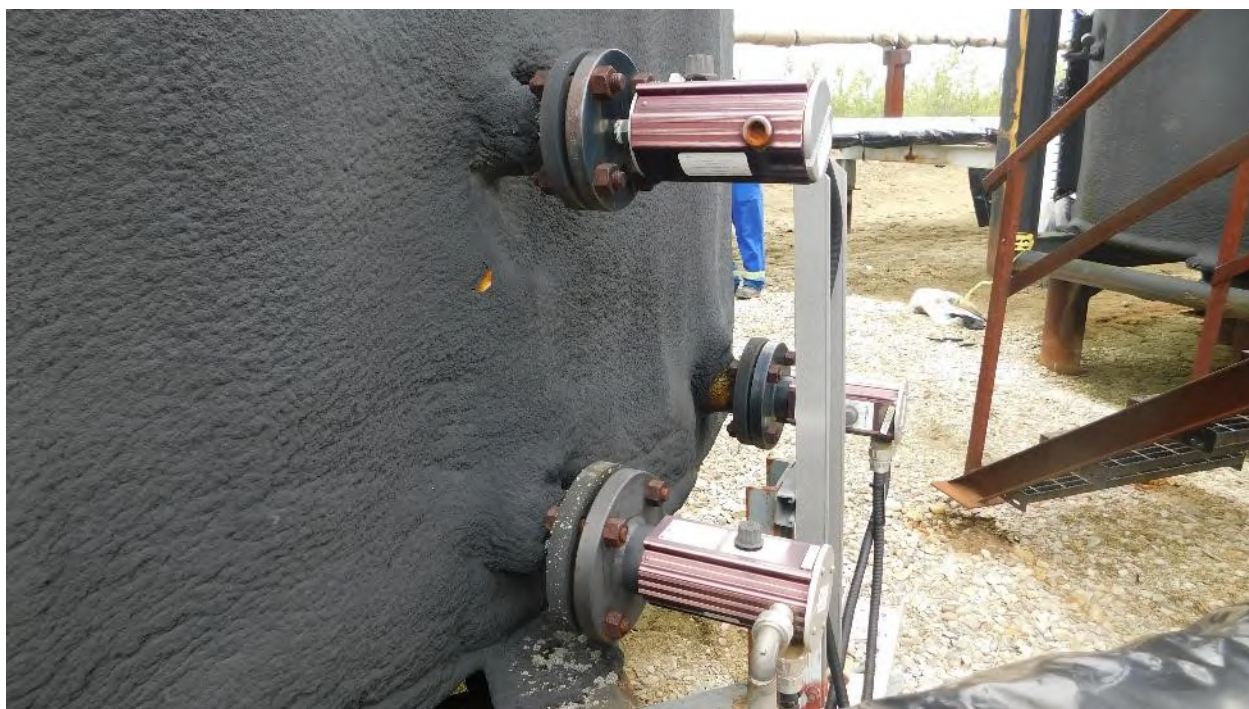
Photograph 50: (3) 2" Instrumentation Nozzles
