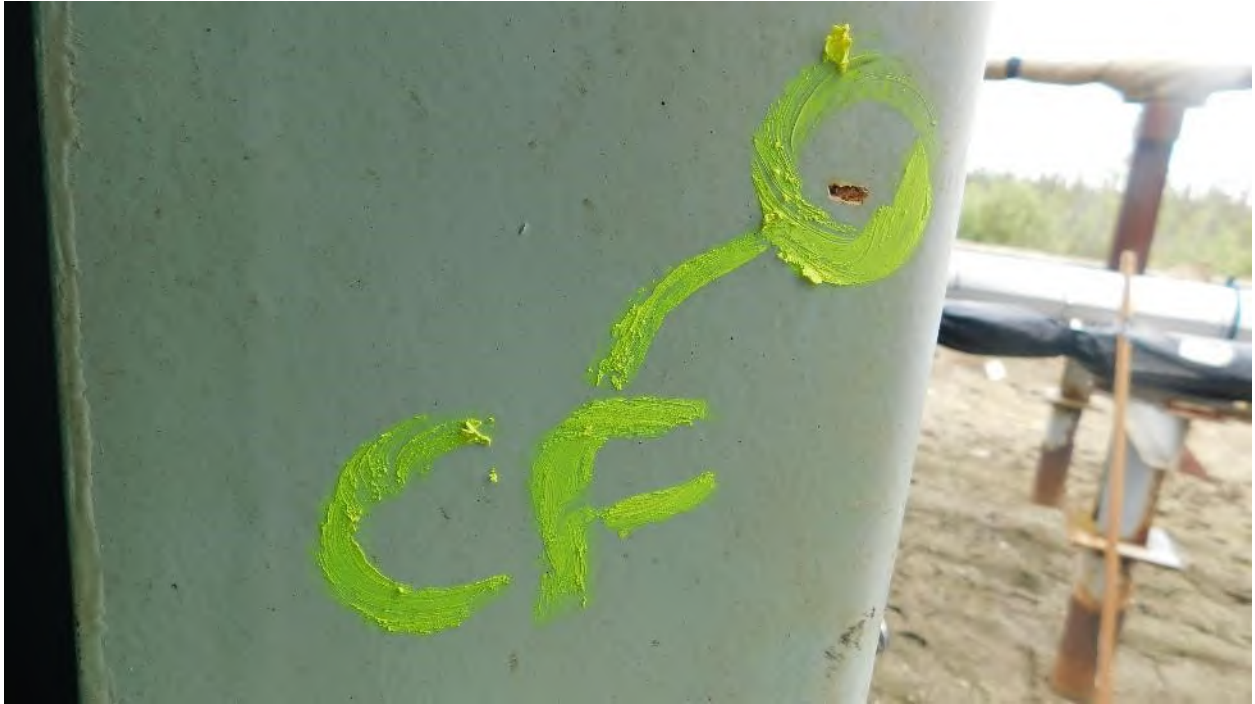
Photograph 55: Manway Coating Failure Detail
