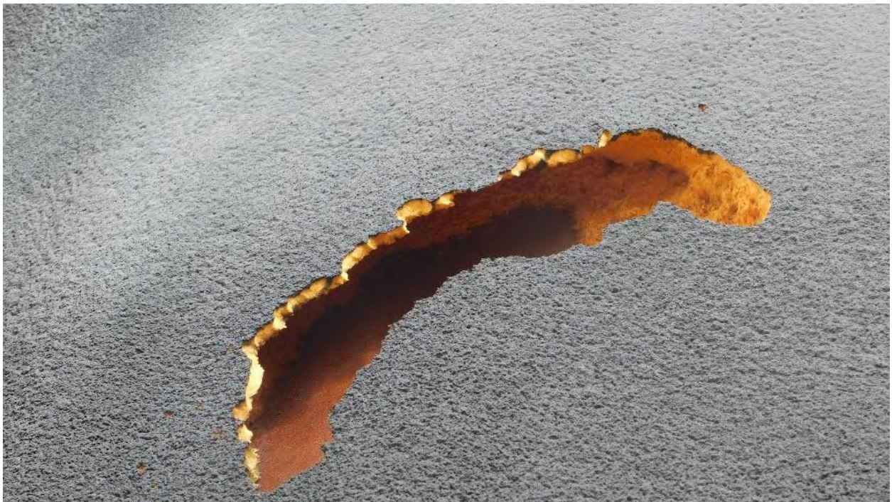
Photograph 35: External Shell Overview – Insulation Damage
