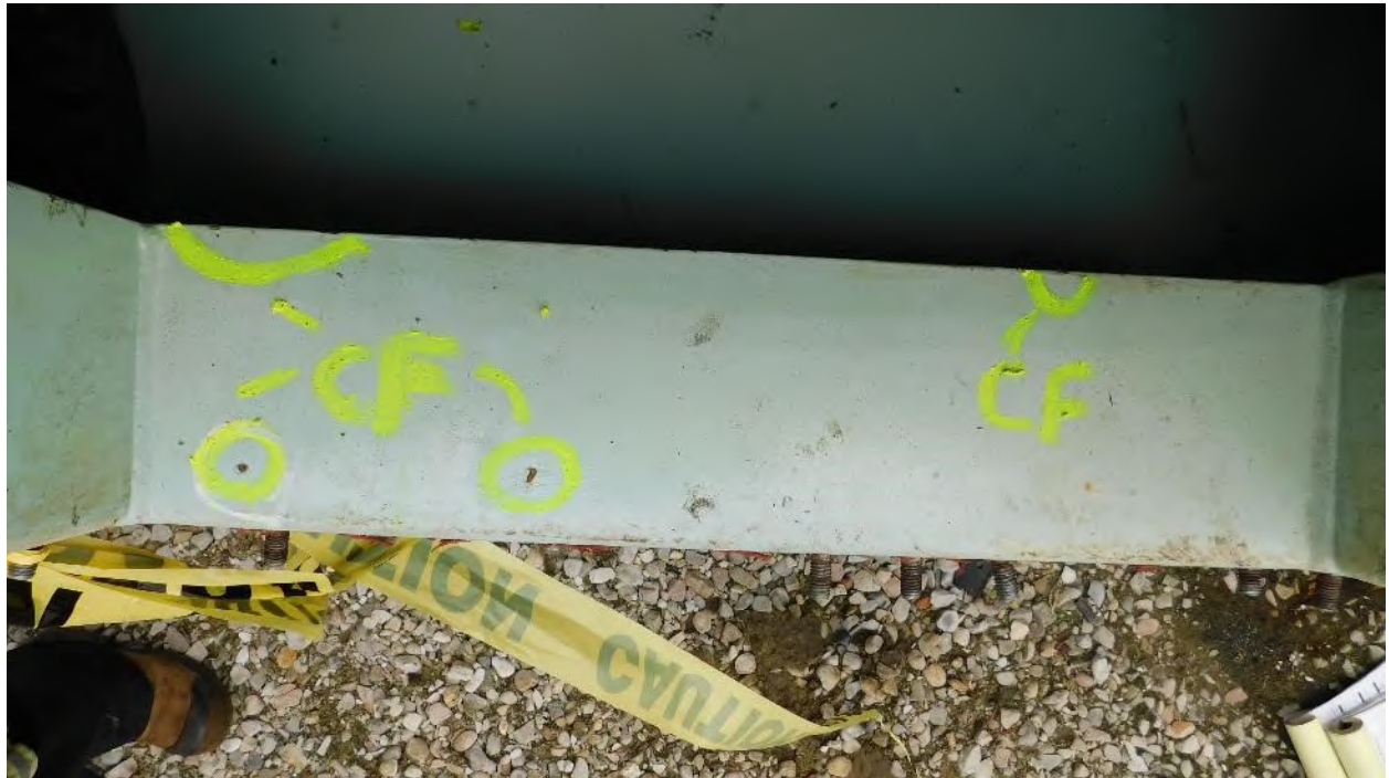
Photograph 53: Manway Coating Failure Overview
