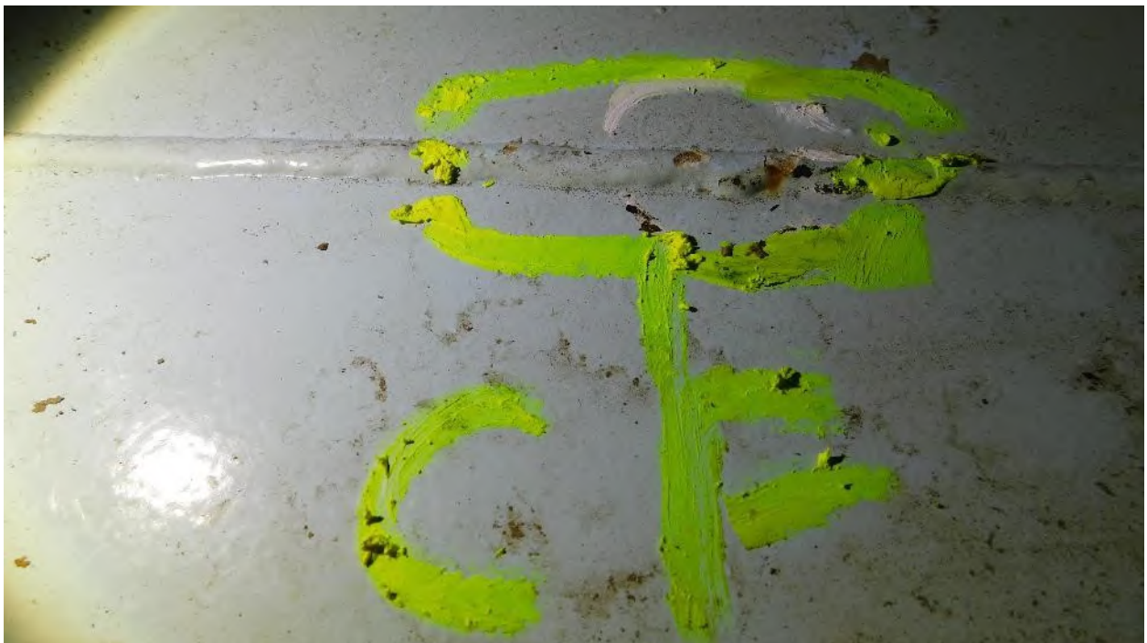
Photograph 26: Bottom Plate Weld Coating Failure Detail
