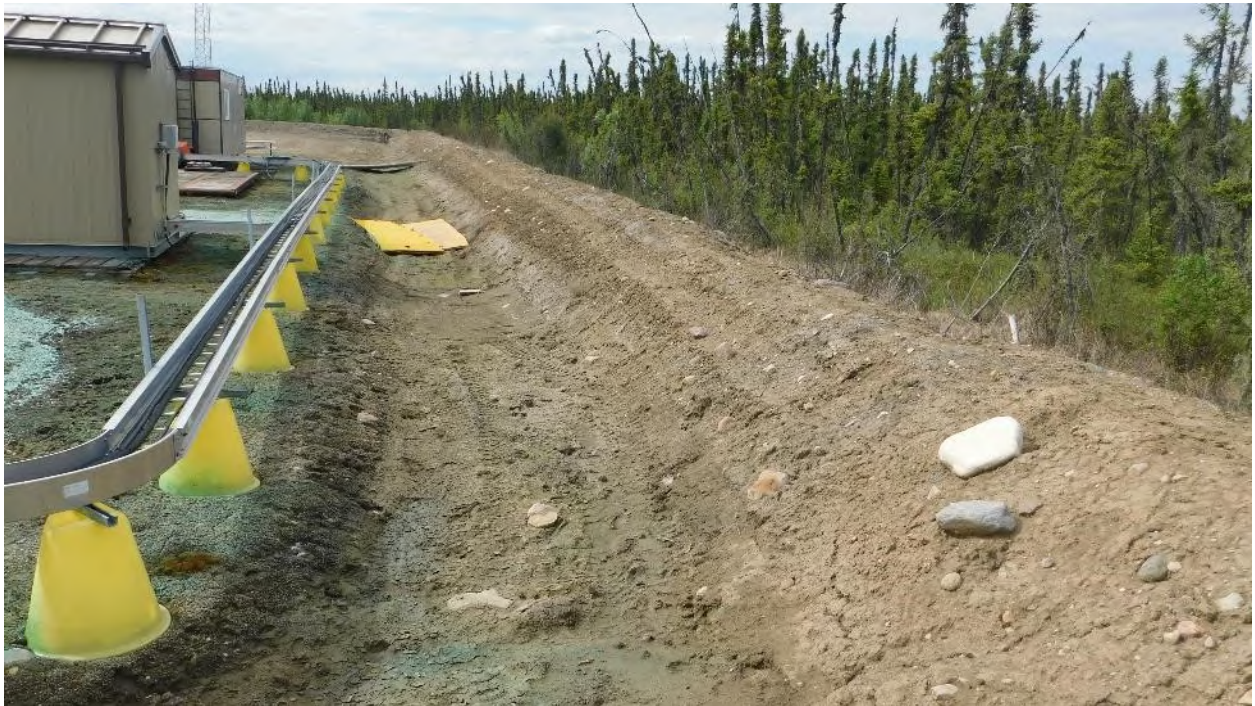
Photograph 8: Secondary Containment Sloped Wall Overview
