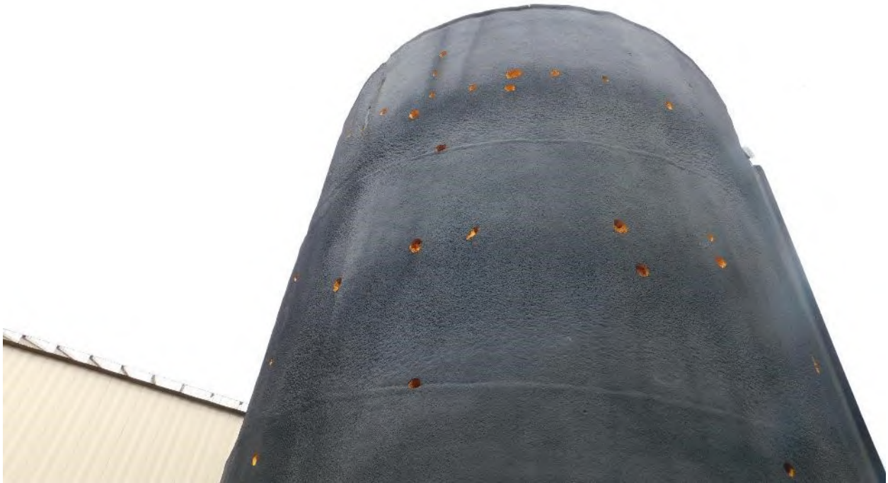
Photograph 36: External Shell Overview – General Minor Insulation Damage
