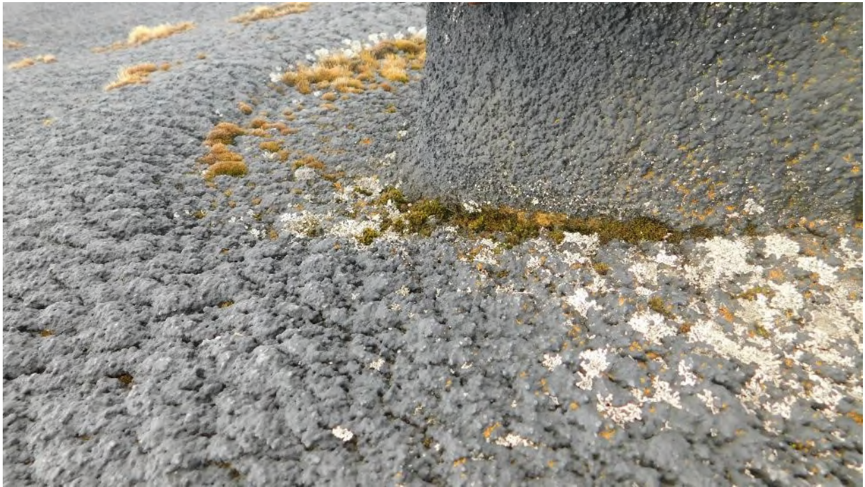
Photograph 68: Gauge Hatch Neck Detail – Moss Growth
