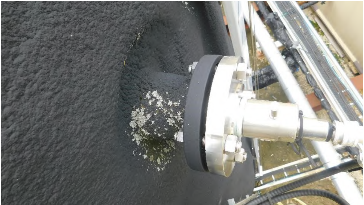
Photograph 51: 2" Instrumentation Nozzle
