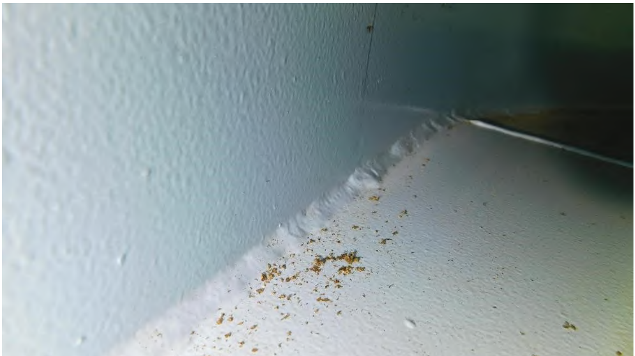
Photograph 32: Internal Shell to Bottom Weld Profile
