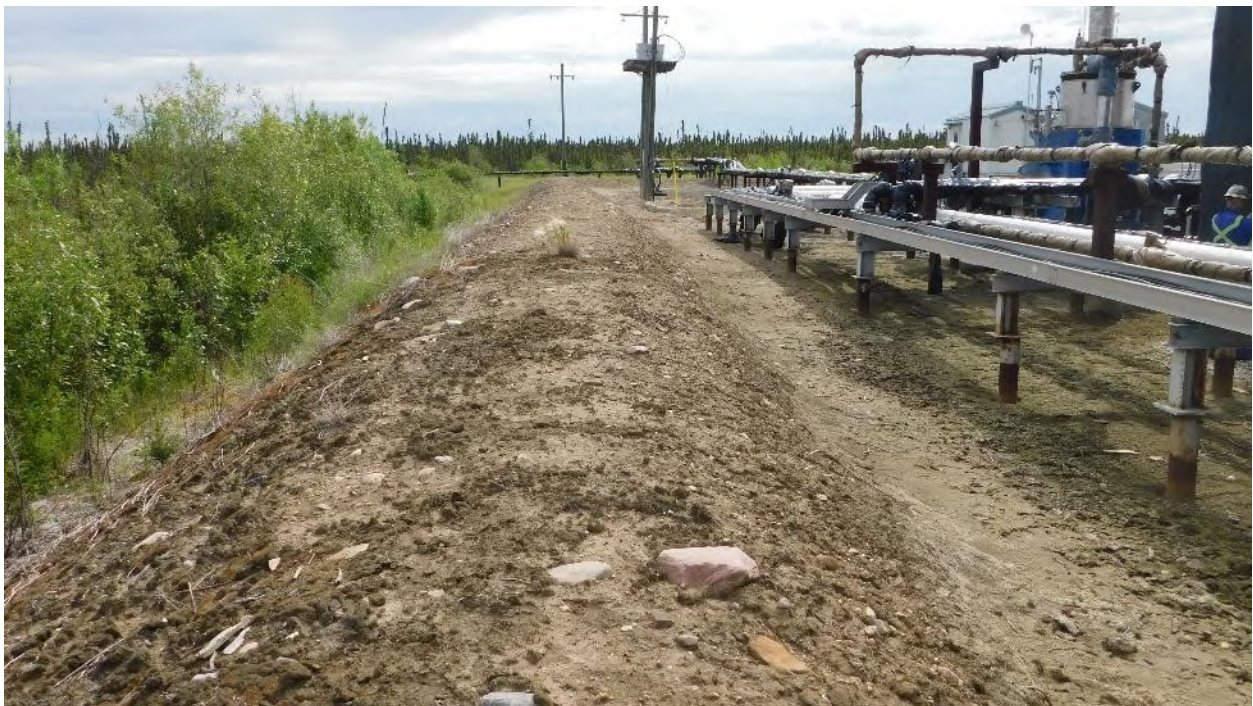
Photograph 7: Secondary Containment Sloped Wall Overview
