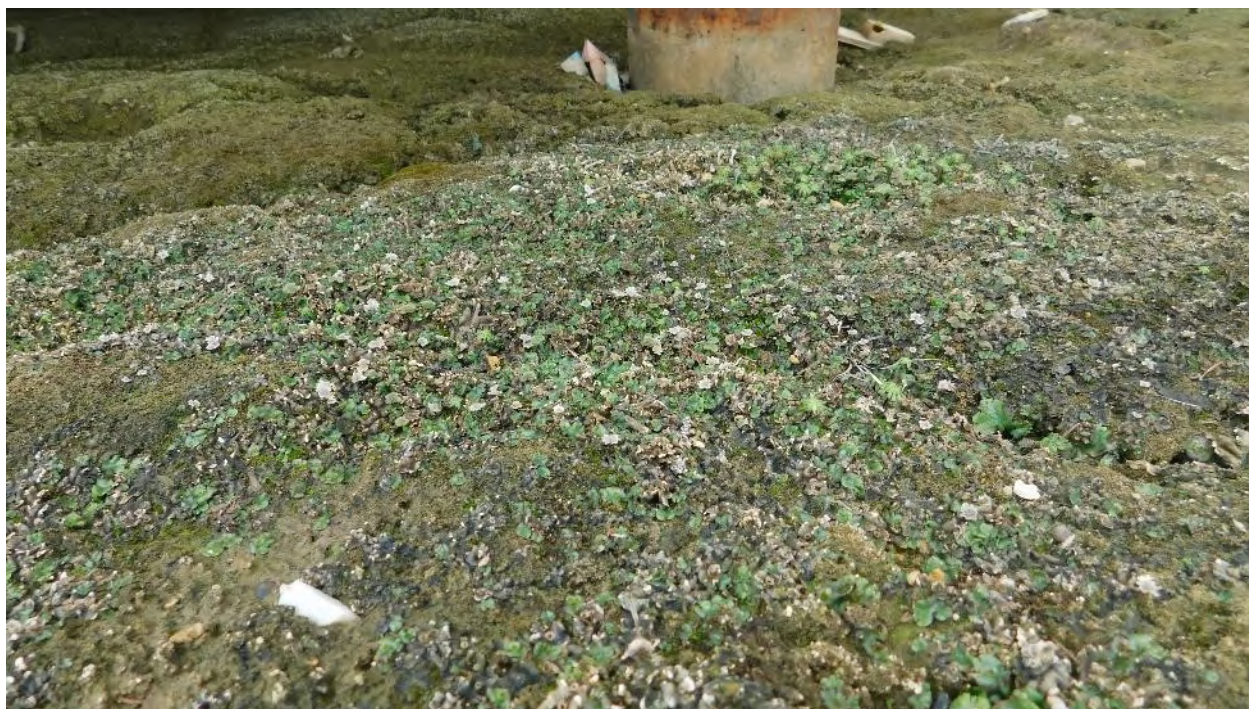
Photograph 12: Secondary Containment Overview – Moss Growth
