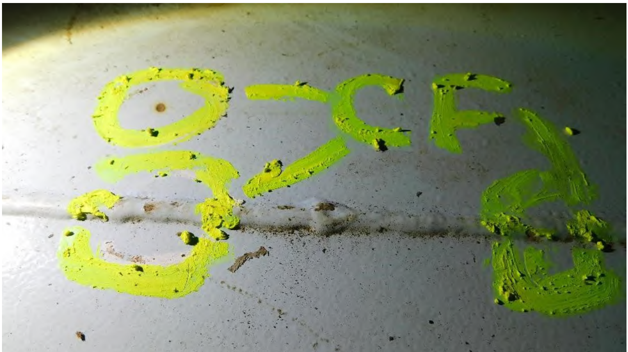
Photograph 30: Bottom Plate Coating Failure Detail
