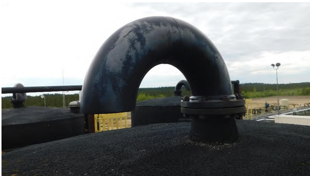
Photograph 71: Gooseneck Vent Overview
