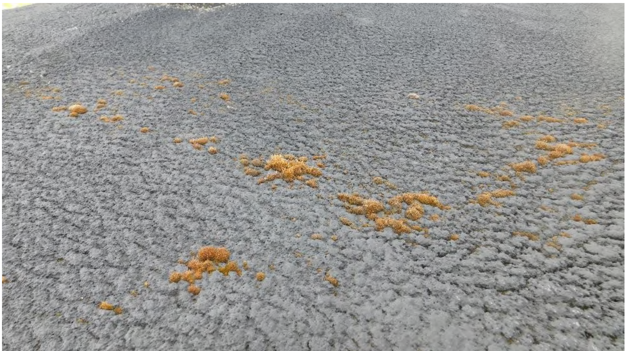
Photograph 69: Fixed Roof – Moss Growth
