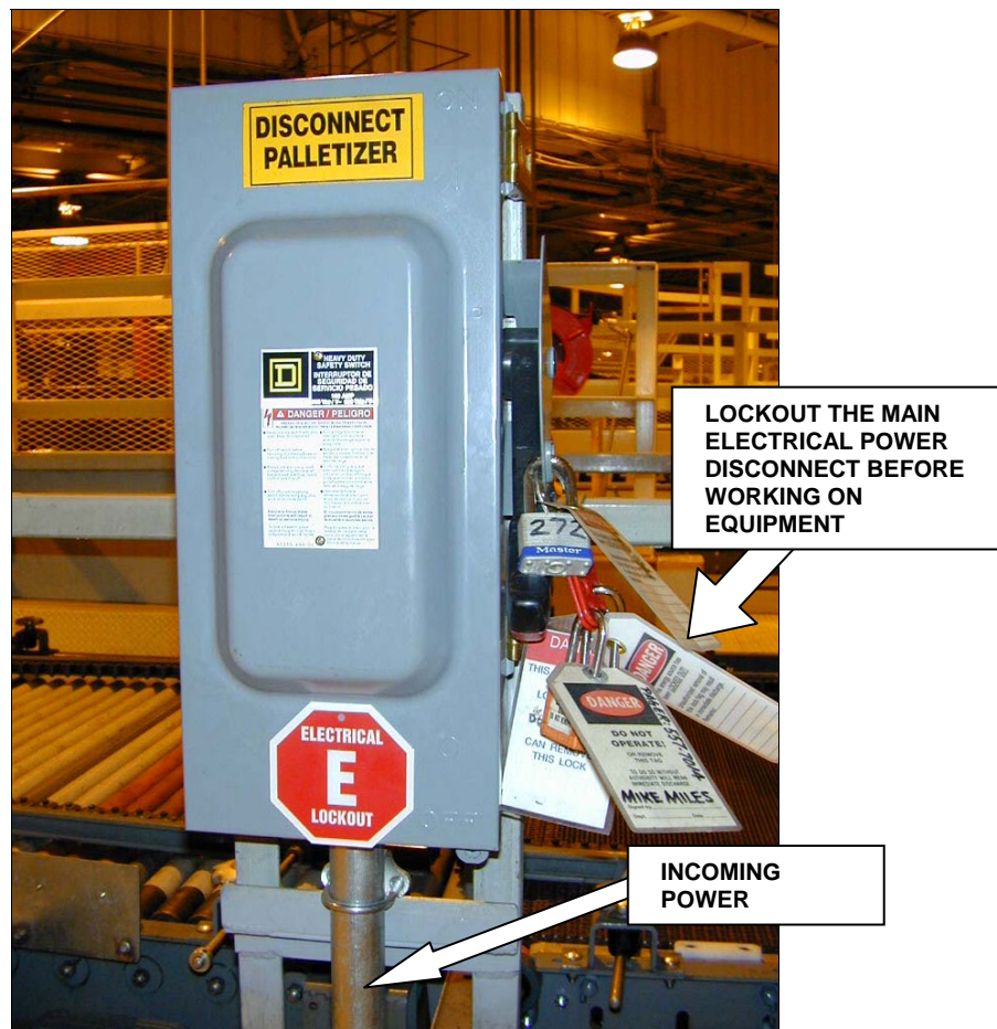
Figure 1-1: Lockout Safety Procedures.
