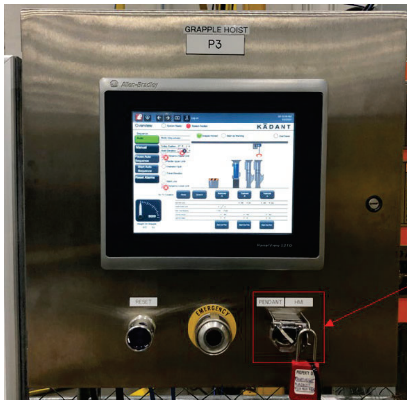
Figure 5-30: P3 HMI Panel Selector Switch
