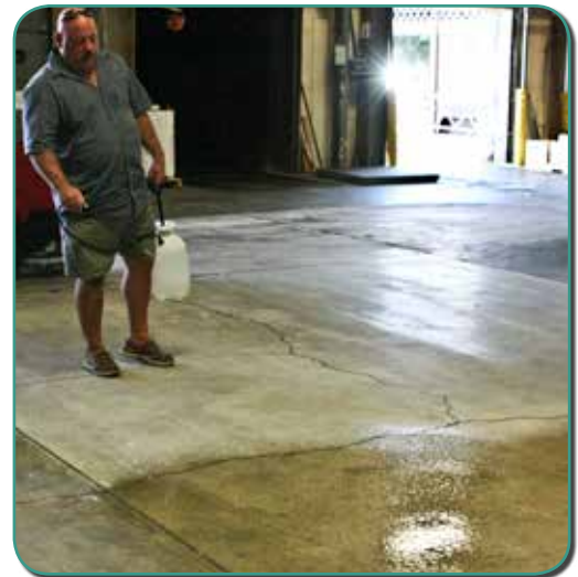
FIGURE 4-A: LAYING DOWN DENSIFIER WITH SPRAY TOOL.
