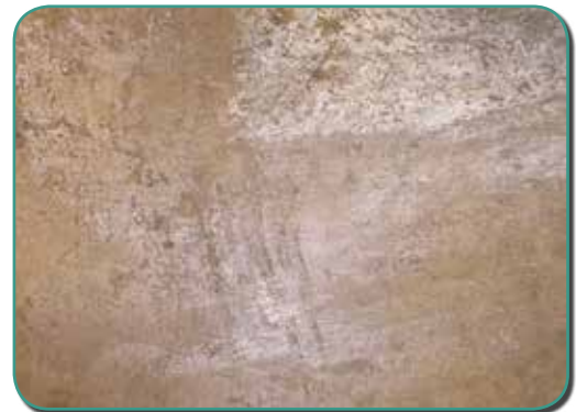
FIGURE 4-B: LEAVING DENSIFIER ON THE FLOOR TOO LONG CAN CAUSE DISCOLORIZATION.
