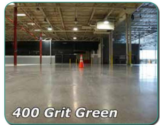
FIGURE 5-A: EITHER STARTING AT THIS POINT TO RETAIN THE POP IN THE SHINE OF THE FLOOR OR THE FLOOR HAS JUST ADVANCED FROM LEVEL 2.
