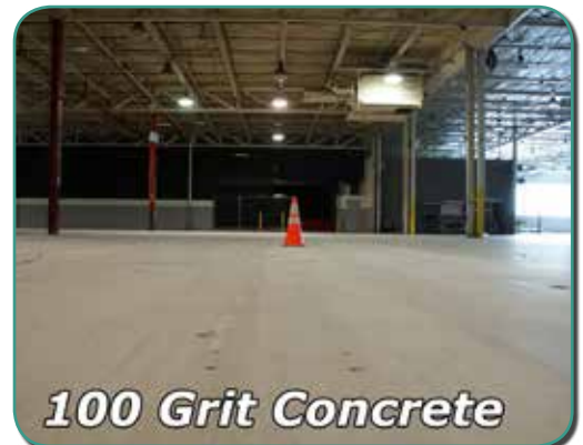
FIGURE 1-E: AFTER 100 GRIT CONCRETE PREP TOOL.
