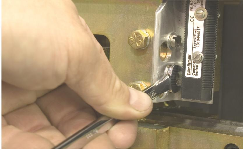
*Figure 60: Removing Photo Eye and Bracket (If Equipped)*
