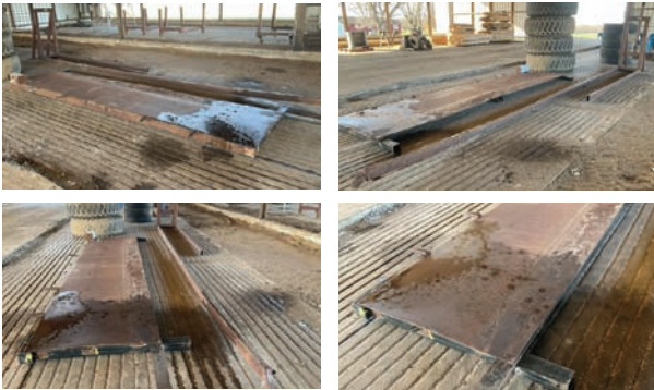
Side Pan 44" x 16' steel side pan, steel 2" x 4" frame.
