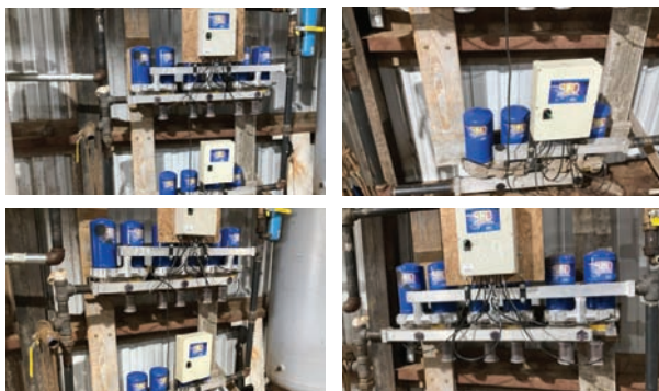
SFD Air Dryer Separator filter dryer, includes connecting pipes.
