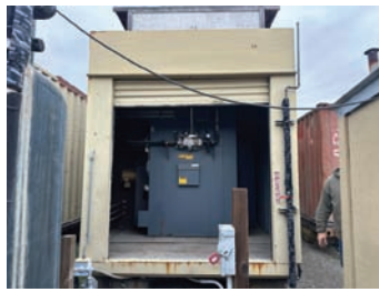
11603 BAKER FURNACE DRY KILNS $15,000.00 Dry Kilns (cream), Conventional Heating System, 600,000 BTU Propane, single phase, 120V control voltage, 3 phase 208V motor voltage, open volume: 672 cubic feet, max operating temperature: 500°F, owners manual included, excellent condition, 2 units available 530-218-4471 RICHMOND, CA
