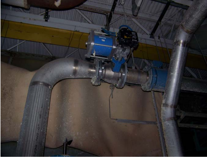
Item 5: Stock flow control valves and flow meters
