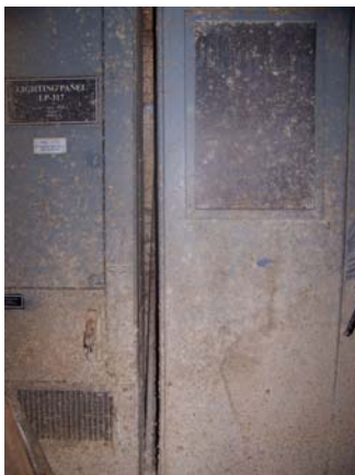
Item 17: 480V lighting switches mounted on drive side of machine
