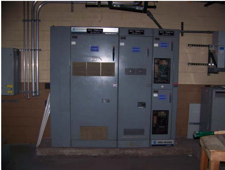
Item 15: Variable Frequency Drive Control Center for Wet Lap
