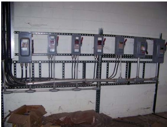
Item 16: 480V switches mounted on wall across from the machine
