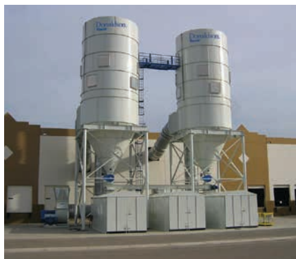
LP on Wood Dust 160,000 cfm (271,784 m 3 /h)
