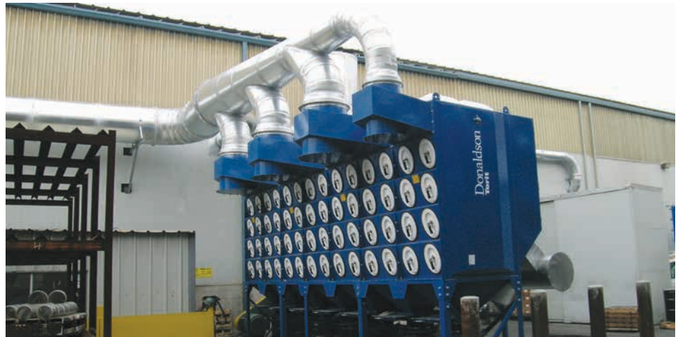
DFO on Grinding 74,000 cfm (125,700 m³/h)
