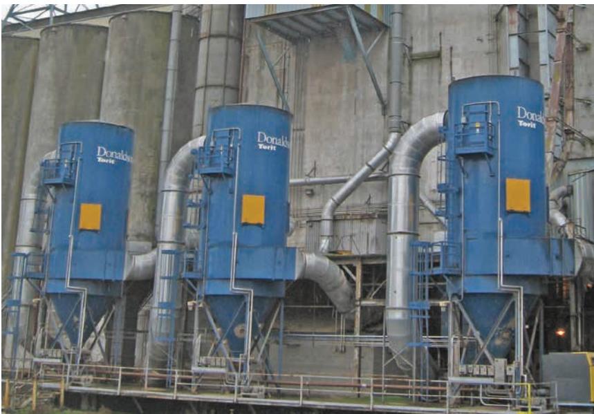
RF - Grain Terminal 61,000 cfm (103,618 m 3 /h)
