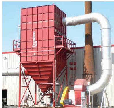
MB on Glass Processing 25,000 cfm (42,466 m 3 /h)
