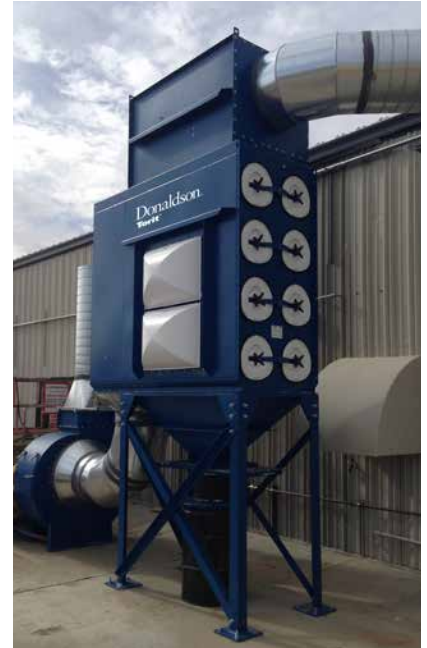
DFO on Plastics Routing 16,000 cfm (27,184 m 3 /h)
