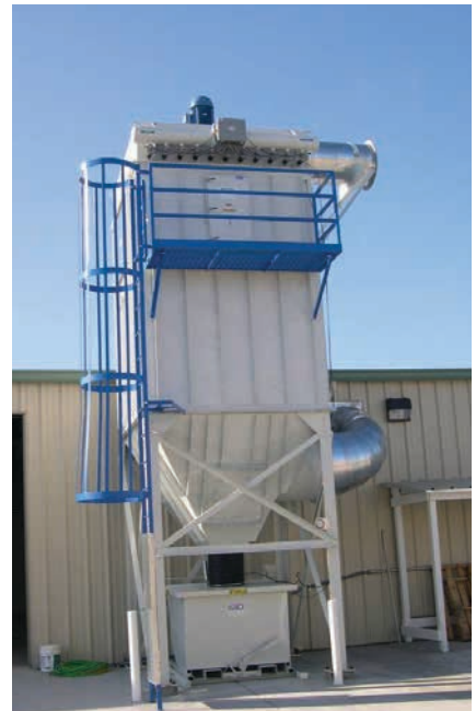
FS on Woodworking 20,000 cfm (33,973 m 3 /h)
