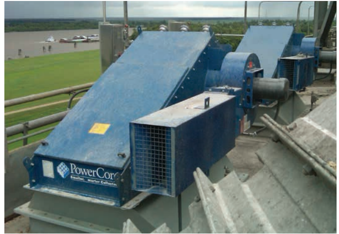
CPV - Direct Bin Venting Distributor Head 2,400 cfm (4,077 m 3 /h)
