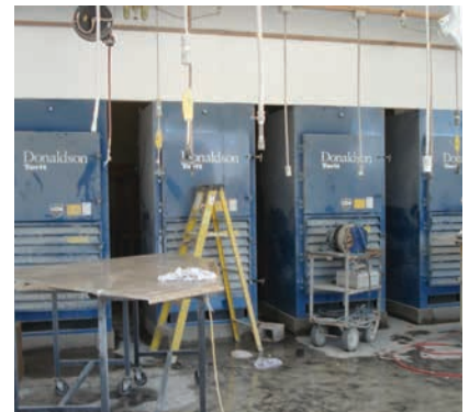
DWS on Granite Finishing 22,000 cfm (37,370 m 3 /h)
