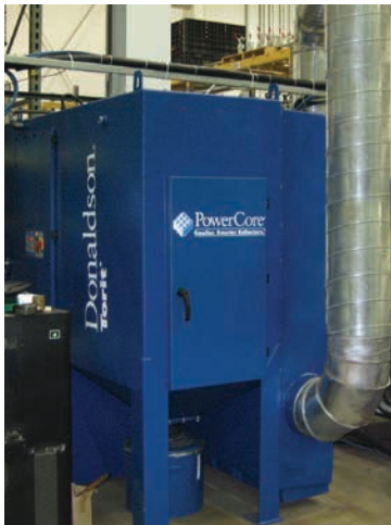
TG on Plasma Cutting 2,300 cfm (3,90 m³/h)
