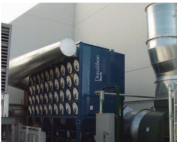
DWS on Custom Hand Grinding 38,500 cfm (65,398 m³/h)
