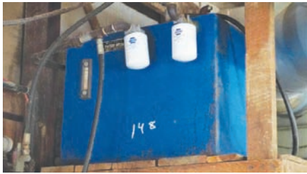
18195 LINE SHAFT $750.00 Hyd tank, and hyd pumps - 3 hyd pumps 260-633-4047
