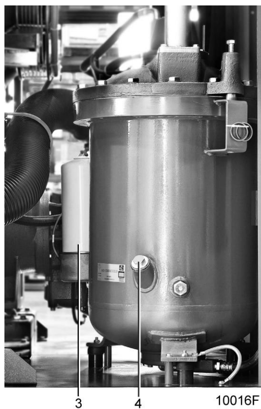
Position of oil filter on G 110 up to G 250
