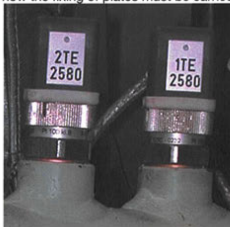
Fig. 18: Sensors with glued on aluminium plate
