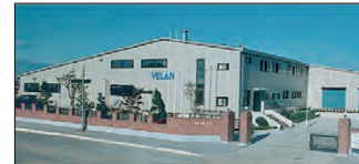
Ansan City, South Korea Velan Ltd., Plant 1
