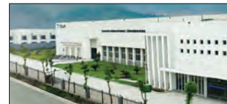
Suzhou, China Velan Valve (Suzhou) Co., Ltd.
