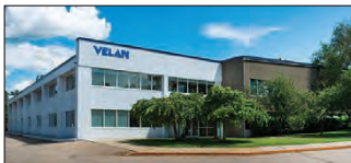
Williston, VT, U.S.A. Velan Valve Corp., Plant 3
