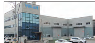
Ansan City, South Korea Velan Ltd., Plant 3
