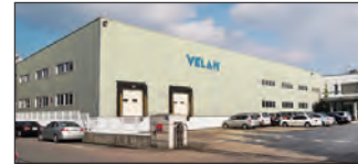
Ansan City, South Korea Velan Ltd., Plant 2
