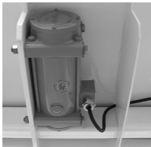
Figure 7-22. Electronic Vibratory Settler
