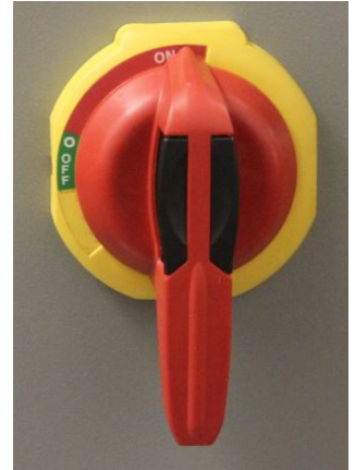
Figure 3-1: Main Power Disconnect Lever
