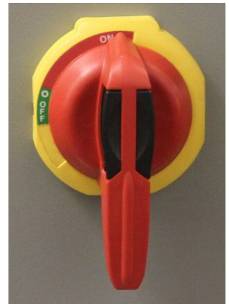
Figure 4-1: Main Power Disconnect Lever
