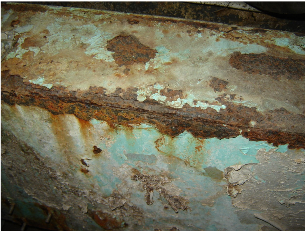
INTERIOR FRAMES CORROSION
