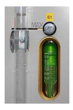
During operation, check the water flow level displayed on the chiller meter
