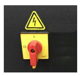
To start up the i-BF; set the Main Disconnect to the ON position, and then press the lit Power ON pushbutton located on the door of the electrical enclosure.
