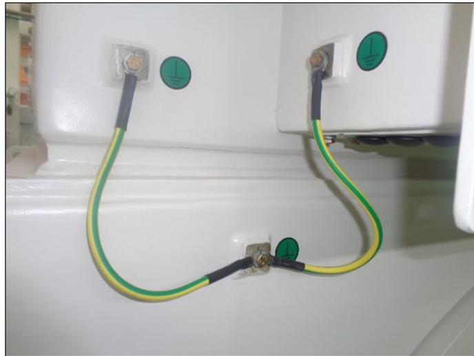
Fig: 5.6-1 – Earthing (Typical Image for reference)
