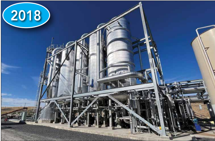
Rosenblad Design Group, Inc. Multi-Effect Evaporator System Manufactured 2018
