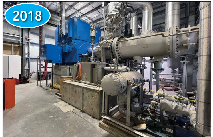
Howden Turbine Generator Twin Series Dual Casing Turbine SST-110 6.9 MW Capacity
