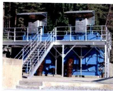
Two AquaDisk® Filters with walkway access.
