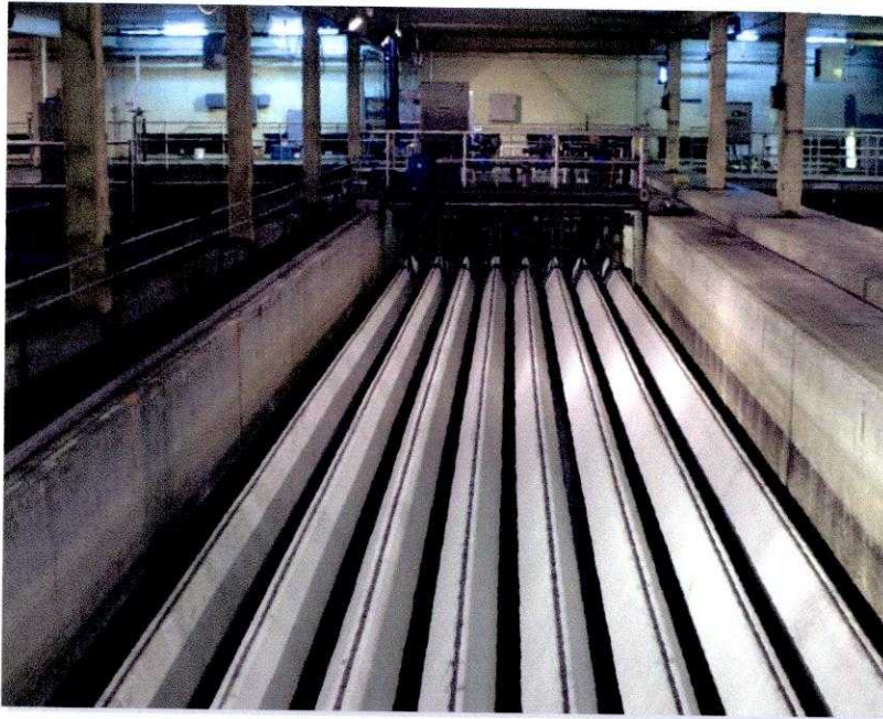
Overview of AquaDiamond® filter retrofitted into a 16' wide sand filter cell.
