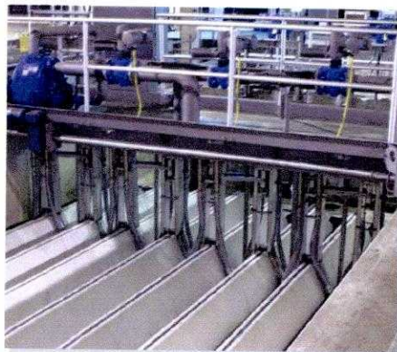
AquaDiamond® backwash assembly and laterals.
