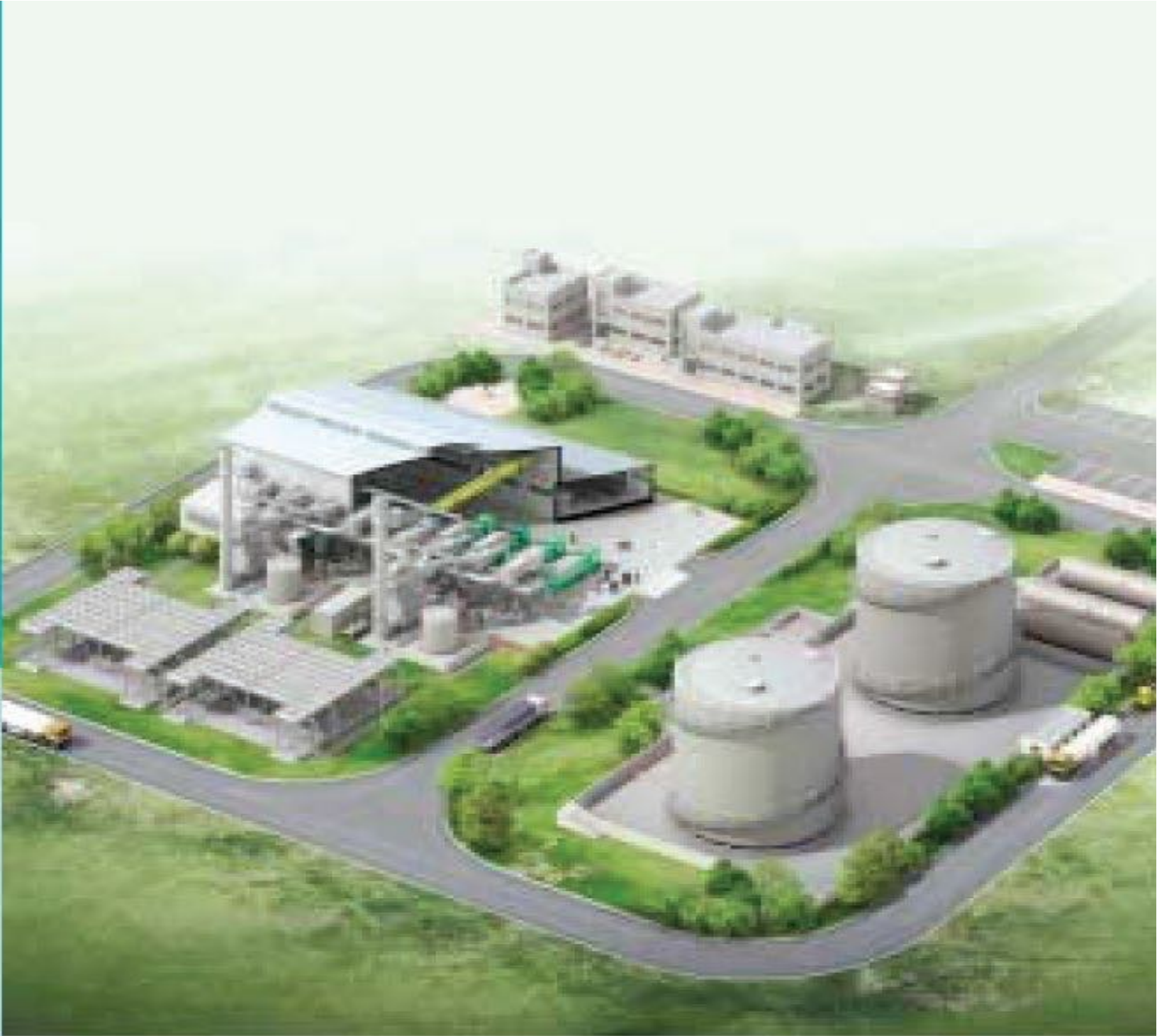
20 MW HiMSEN Engine Diesel Power Plant (9H25/33 X 8 Sets)
