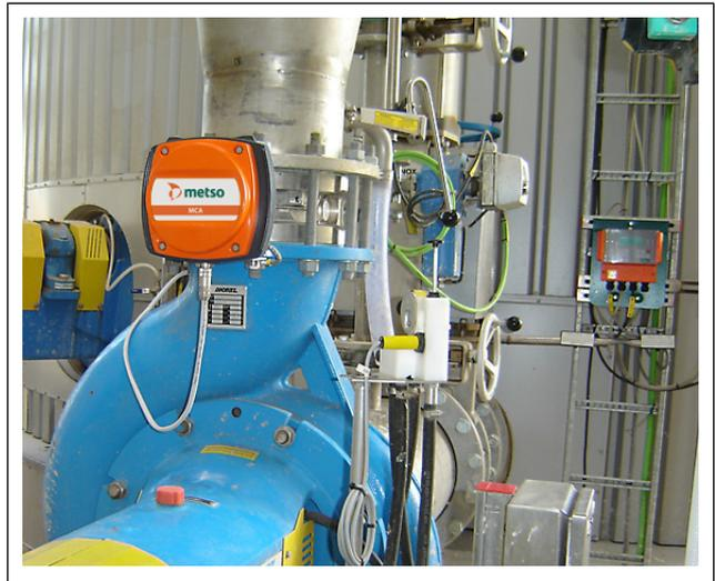
*Fig. 6. Metso MCA-FT installation directly after a pump.*
