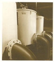
The recovery system is comprised of three WWF's utilizing 165-mesh screens to process a cumulative total of 1600 gpm.
