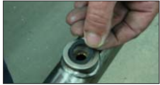
Fig. 1, place the gasket
