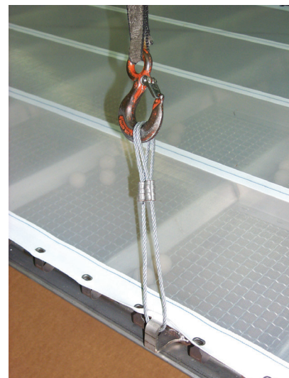
3.3 Screen frame removal using lifting hooks and overhead hoist
