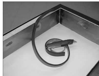
3.28 Installation of Top Cover Seal
