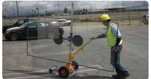
Extension arm available for lower glazing work and glass balustrading.
