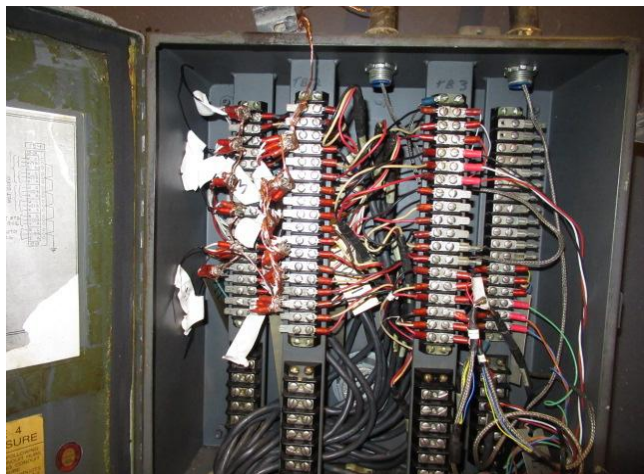
Stator RTD's disconnected, labeled and tested.
