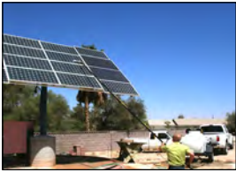
SOLAR PANEL CLEANING
