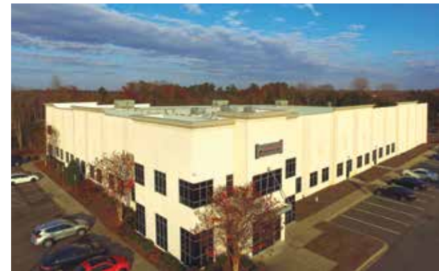
Bradman Lake's new purpose-built freehold manufacturing facility, Rock Hill, SC, USA.
