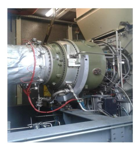
Unit was originally installed in 1995, stopped in 2000, re commissioned by us in 2006 and has been serviced by us since then. Received its last overhaul in 2012 including new Siemens supplied HP rotor blades. (expected lifetime is 24000 operating hours)
